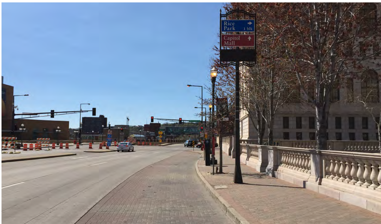
Existing conditions on Kellogg Boulevard.
