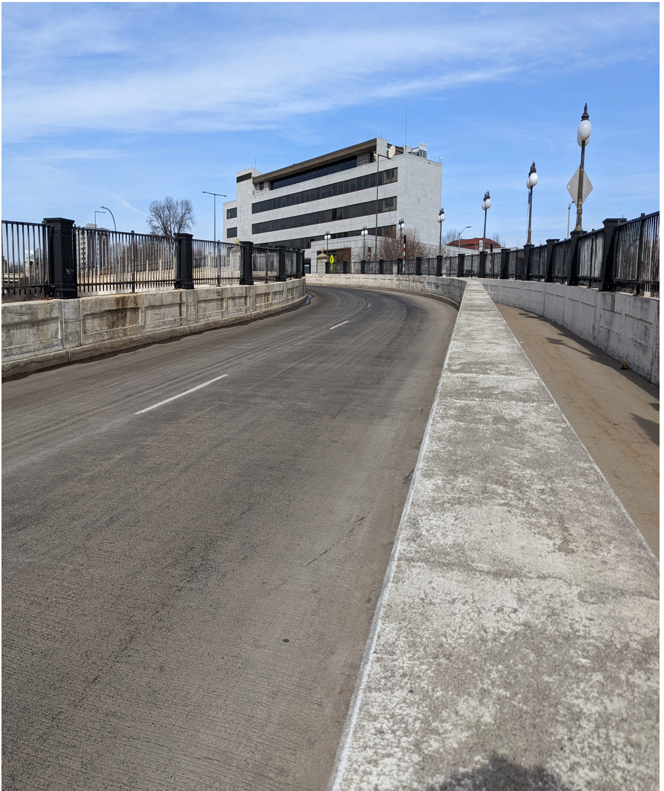
Existing Condition photo
