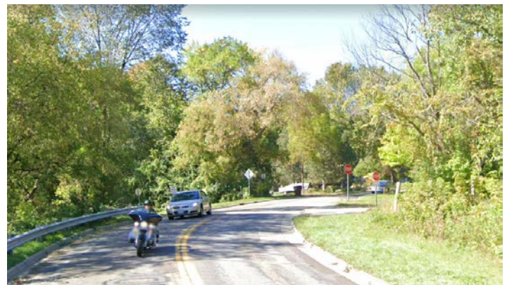
Unsafe trail crossing; limited sightlines and signage (looking northwest)
