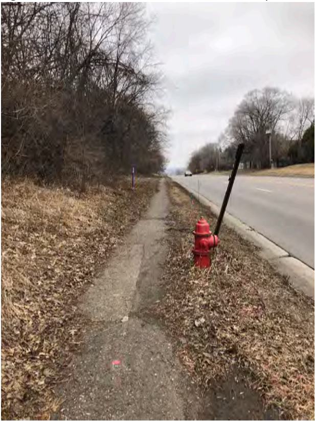
Fig 2. W 94 th to W 98 th Street, West side – Examples of narrow path, deteriorated pavement, and clear zone obstructions
