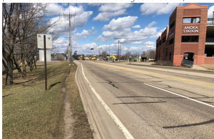
Existing Conditions (4th Avenue north of Pierce Street- facing northbound)
