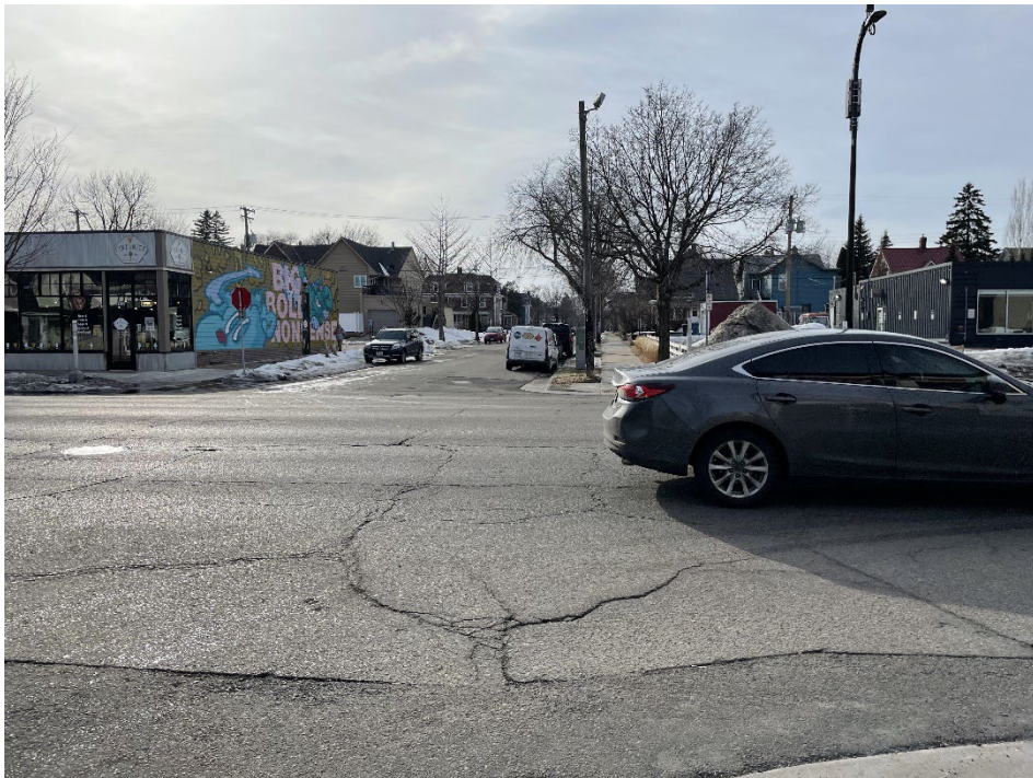
(Left) The intersection of 27 th and Lyndale Ave, is a barrier to pedestrians and cyclists due to high speeds and long crossing distances. Throughout the corridor, much of the roadway is experiencing significant cracking and pavement markings are worn.
