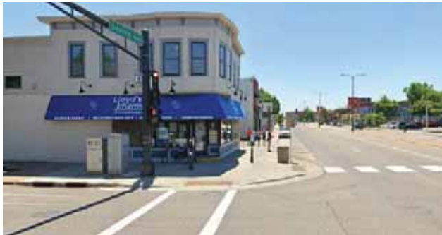
Curb retrofit on Snelling Avenue, Saint Paul, MN; Source: Google
