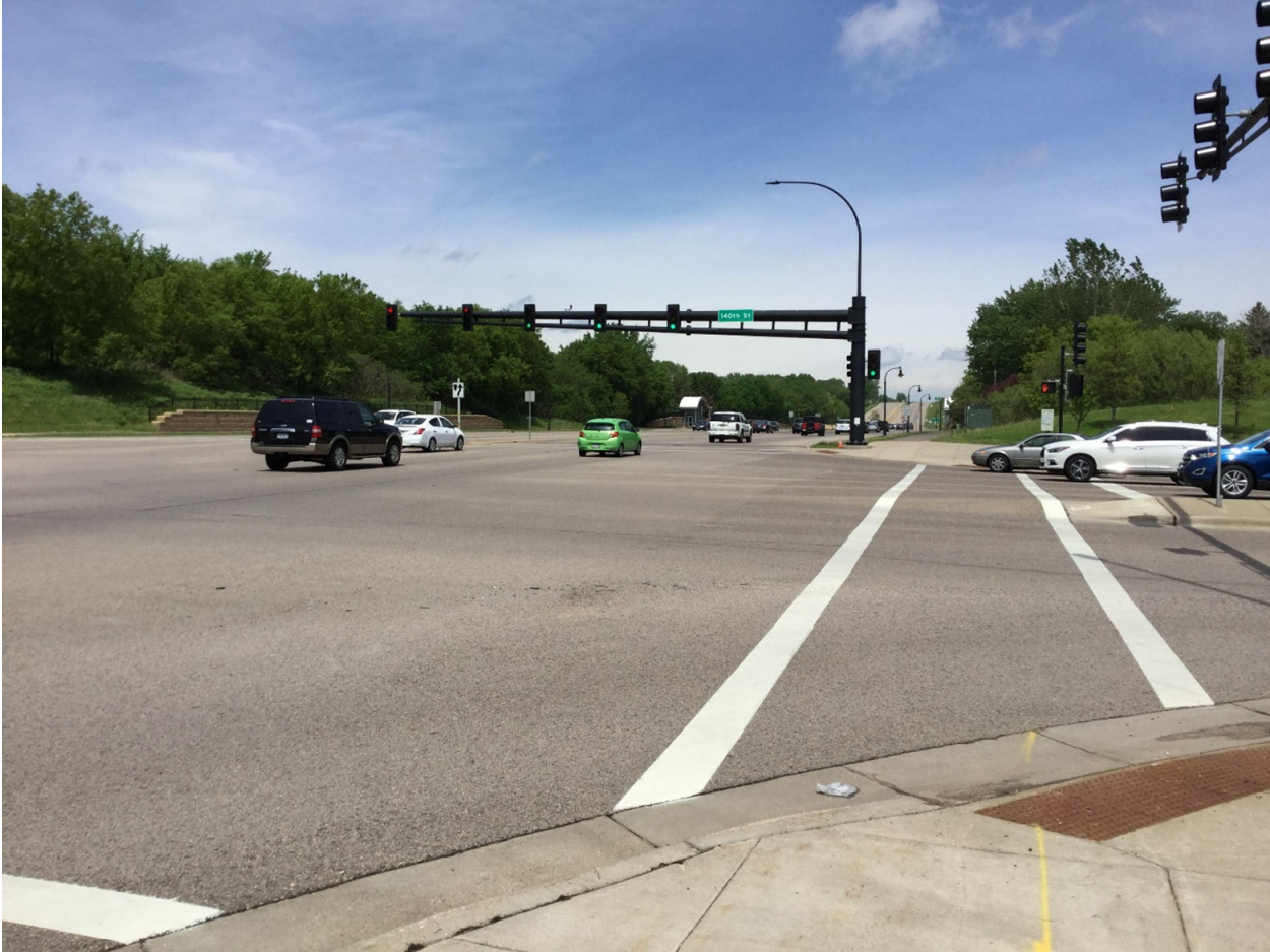
Existing Conditions: Cedar Avenue at 140 th Street, facing north towards the project site.
