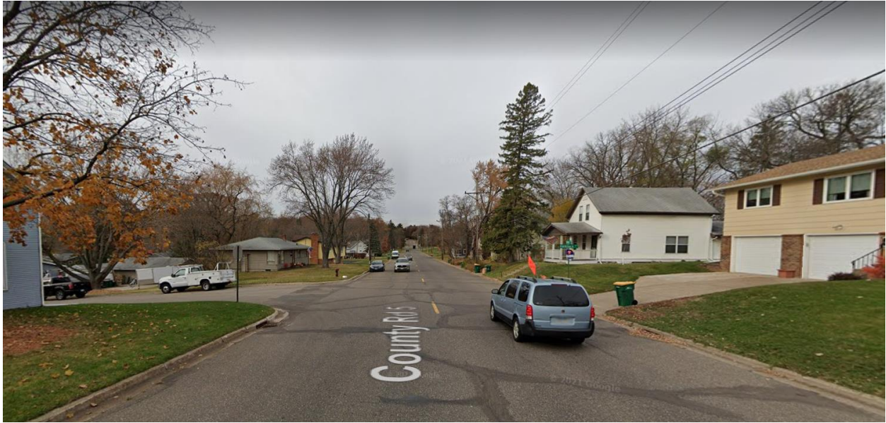
Image 4. CSAH 5 at Owens Street, facing west
