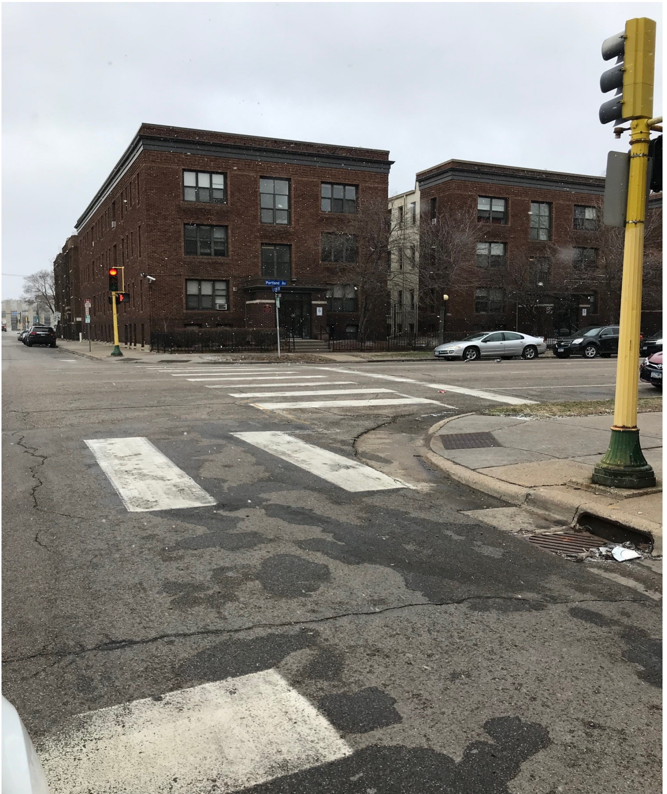
Existing conditions photo
