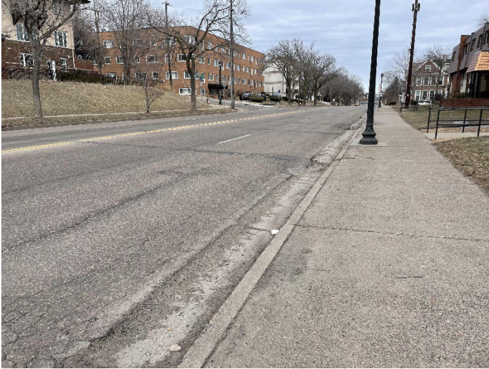
Overview of the existing undivided 4-lane configuration, which creates difficult midblock crossings for the 0.5 mile stretch from CSAH 22 to Blaisdell Ave.
