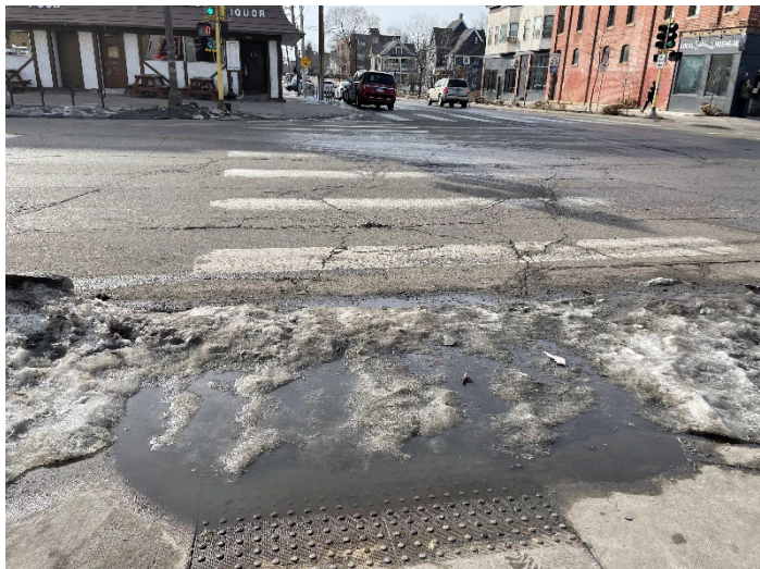
Even where truncated zones are present, ice and snow, as shown above at the 26 th St. intersection, pool at crossings due to drainage issues, creating barriers to accessibility.
