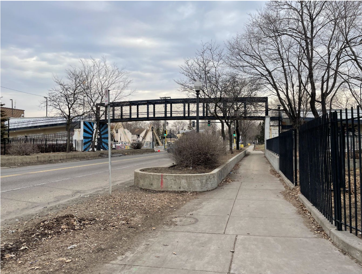
(Above) The crossing at the Little Earth development is both at-grade and grade separated through a pedestrian bridge. As shown above, the pedestrian bridge can block sightlines for the at-grade crossing signal.
