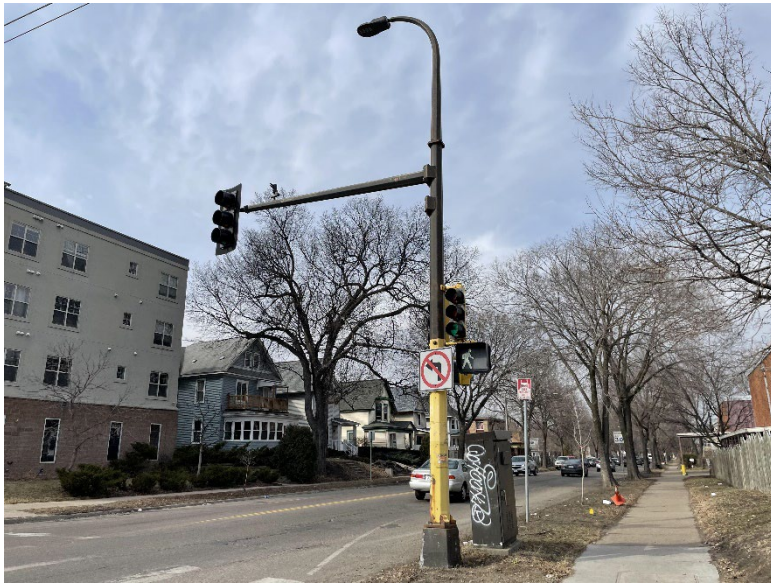
Many signals are aging and are in need of replacement, such as this signal at the 28 th St and Cedar Ave intersection which was originally constructed in 1966.
