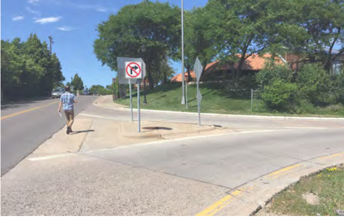
Figure 1.10 Example of discontinuous pedestrian facilities and unmarked crosswalks within the District.
