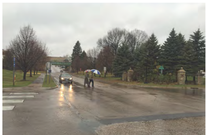
Figure 1.5 Existing condition of Eden Avenue at Arcadia Avenue, showing a lack of pedestrian crossing and sidewalk facilities. From the design team's site visit, November 2015.
