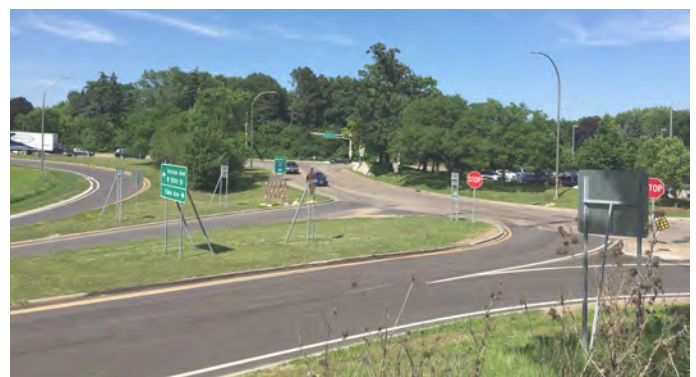
Figure 3.38 Existing redundant ramps and under-utilized space on east side of Highway 100.
