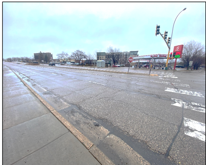
VIEW: Looking northeast at the signalized Edin Ave intersection April, 2022
