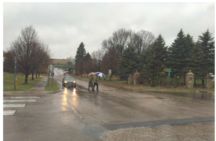
Figure 1.5 Existing condition of Eden Avenue at Arcadia Avenue, showing a lack of pedestrian crossing and sidewalk facilities. From the design team's site visit, November 2015.
