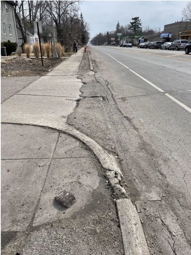
Cyclist utilizing the sidewalk, leading to potential user conflicts. Looking south at the 67 th St intersection.
