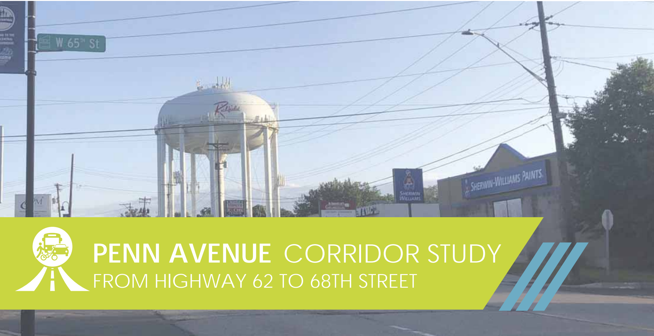
Penn Ave looking north from 65th Street
