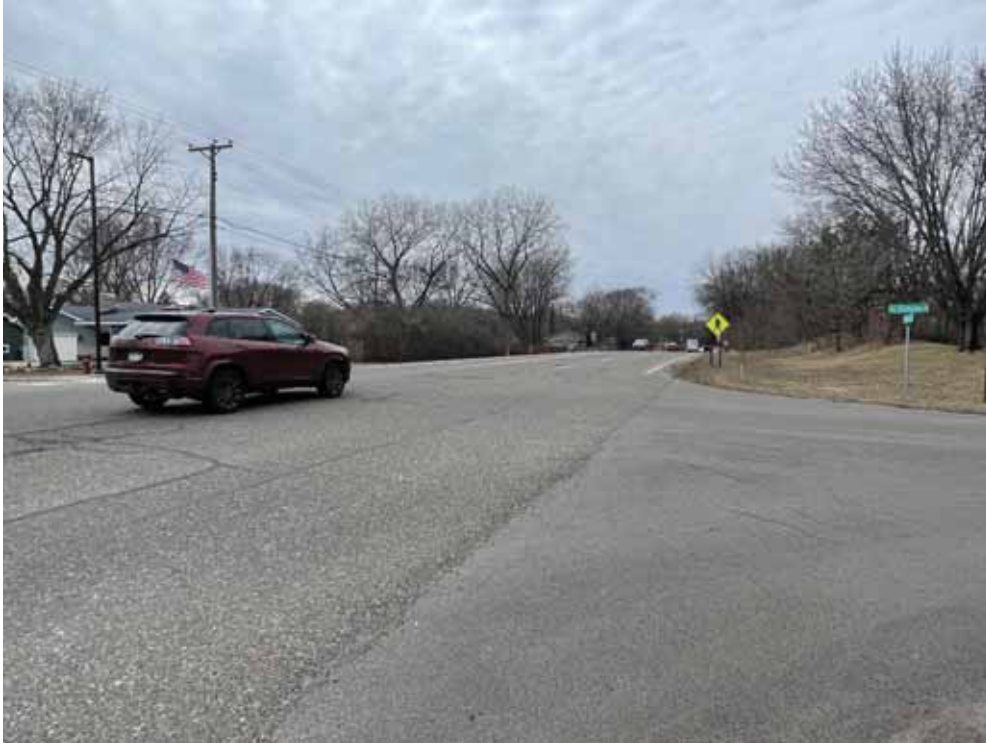
Bypass lane and pedestrian crossing at the Dayton River Rd and Sunrise Ln, looking northwest.
