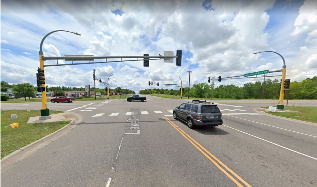
CSAH 9 looking south from the northern extent of the project area.
