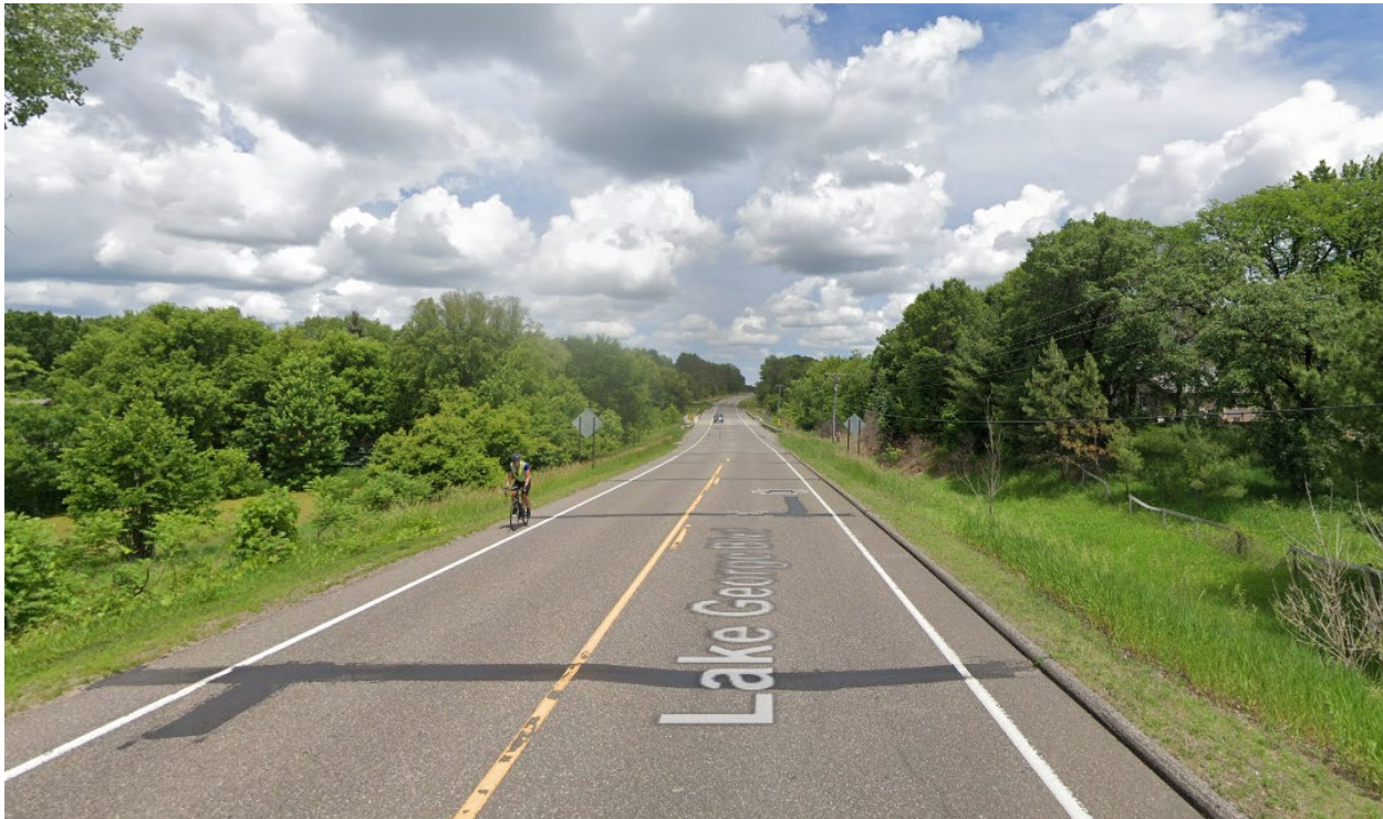
Documentation of narrow shoulders in project area.
