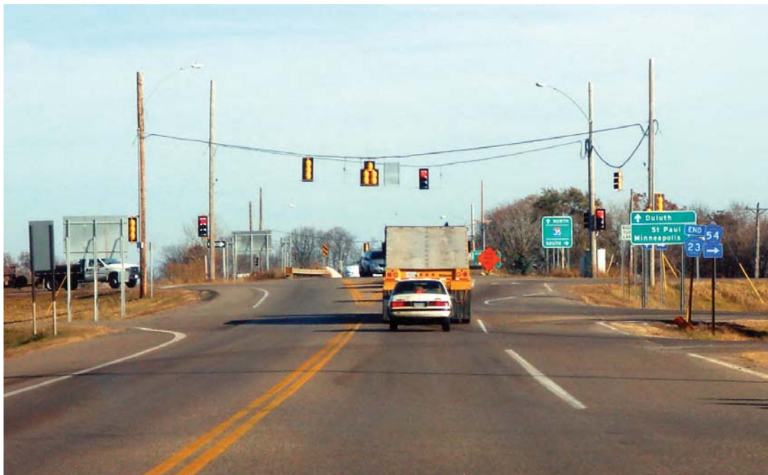
Intersection in Anoka County (Source: Anoka County)
