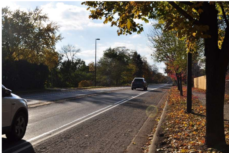
Figure 4 – Cedar Lake Road looking west. Parking lanes, no sidewalk on left side of roadway, no bikeway, pavement condition in need of repair
