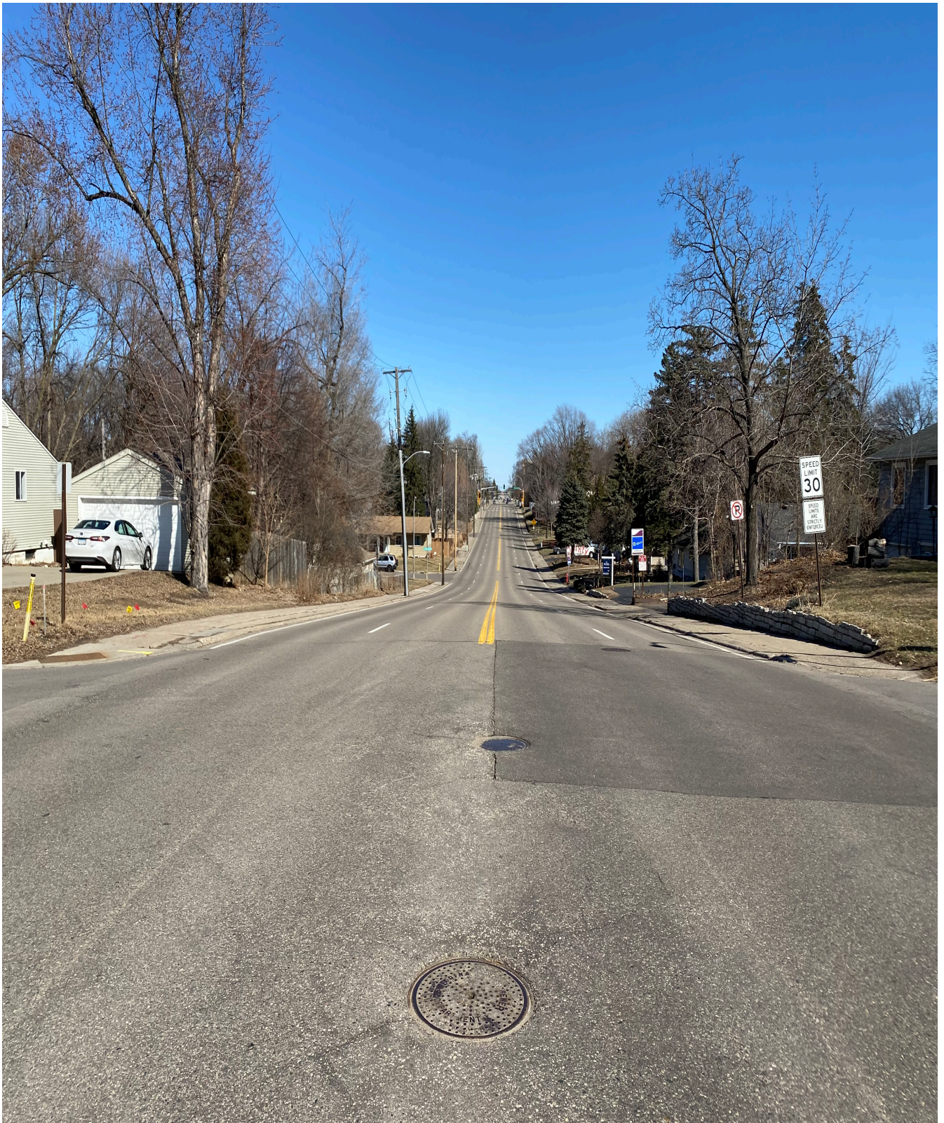
Existing site condition photo
