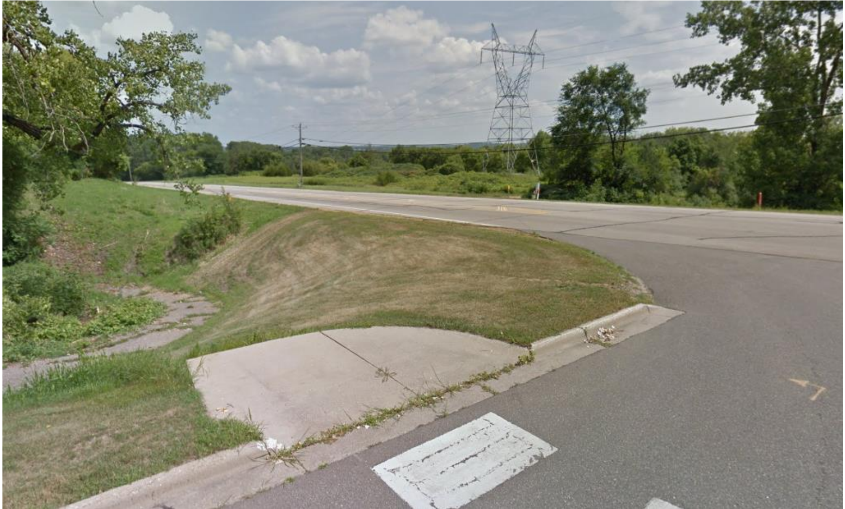
CSAH 10 Existing Conditions – Existing overgrown pedestrian underpass at Ridge Lane
