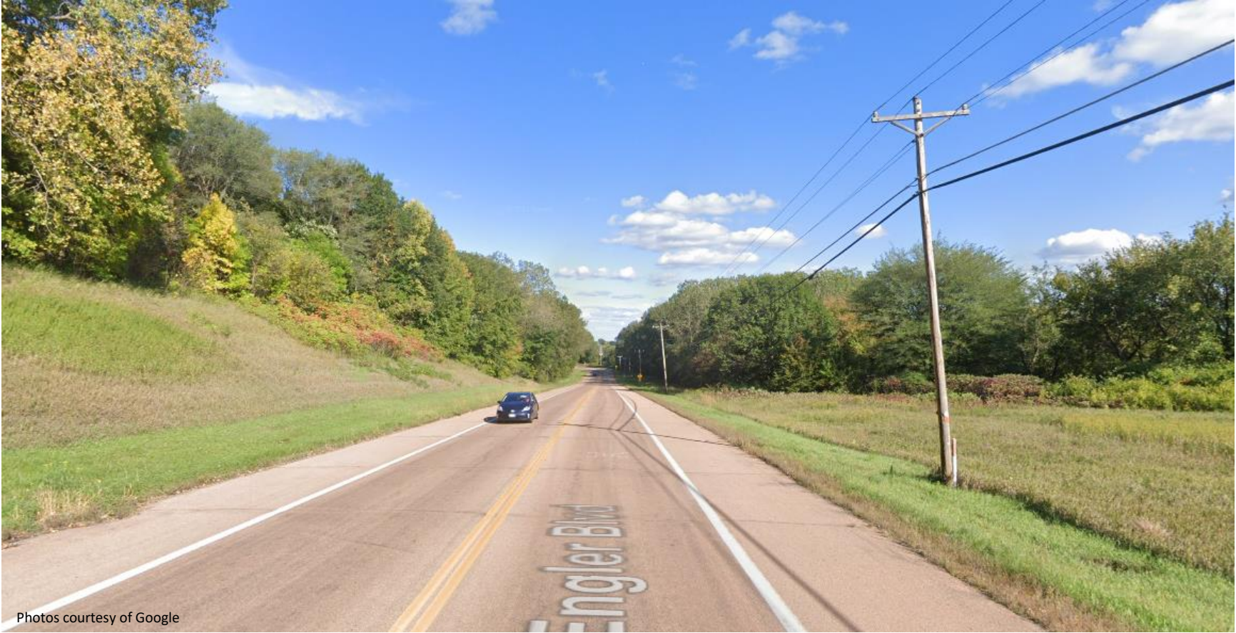
CSAH 10 Existing Conditions – Looking east at Ridge Lane
