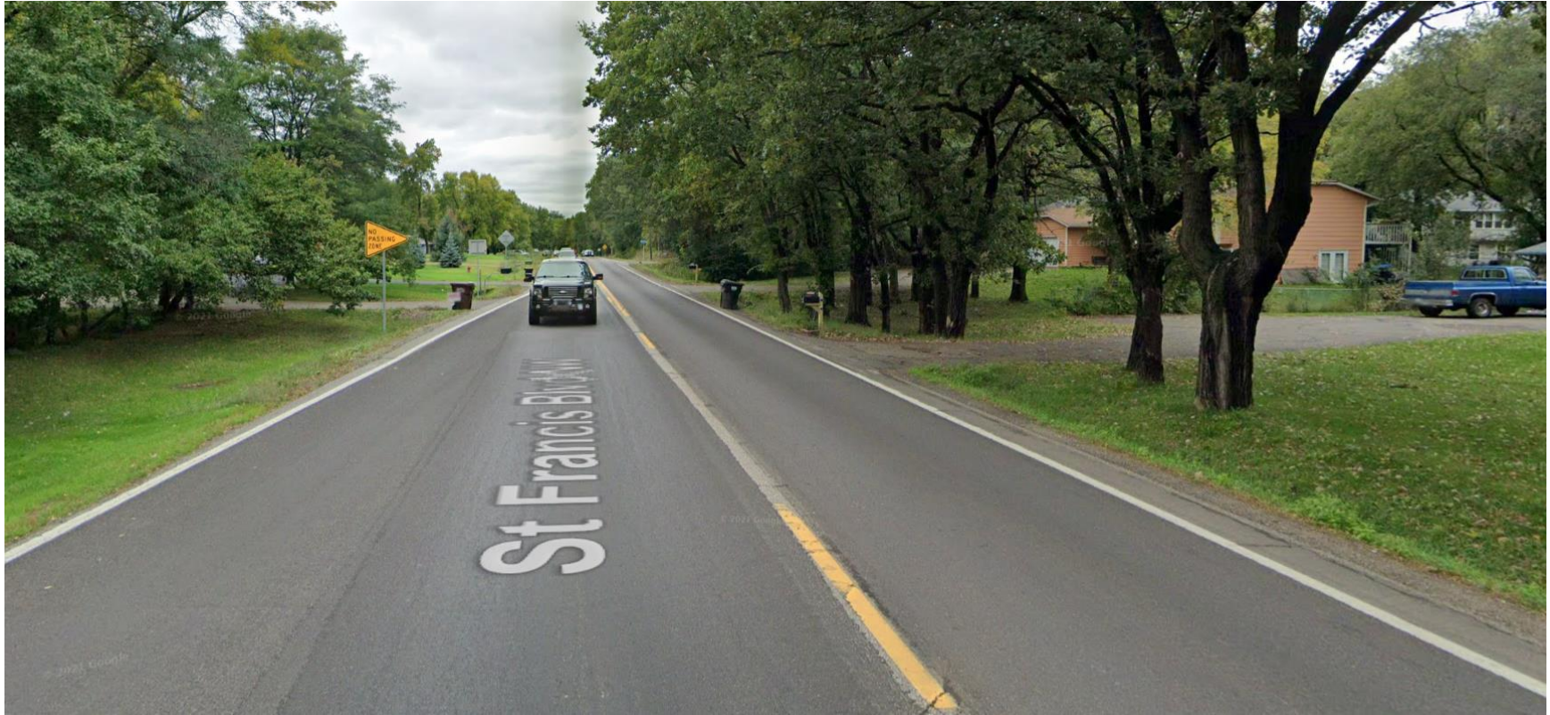
TH 47 Corridor Improvements – Existing Conditions: At McKinley Street, looking north
