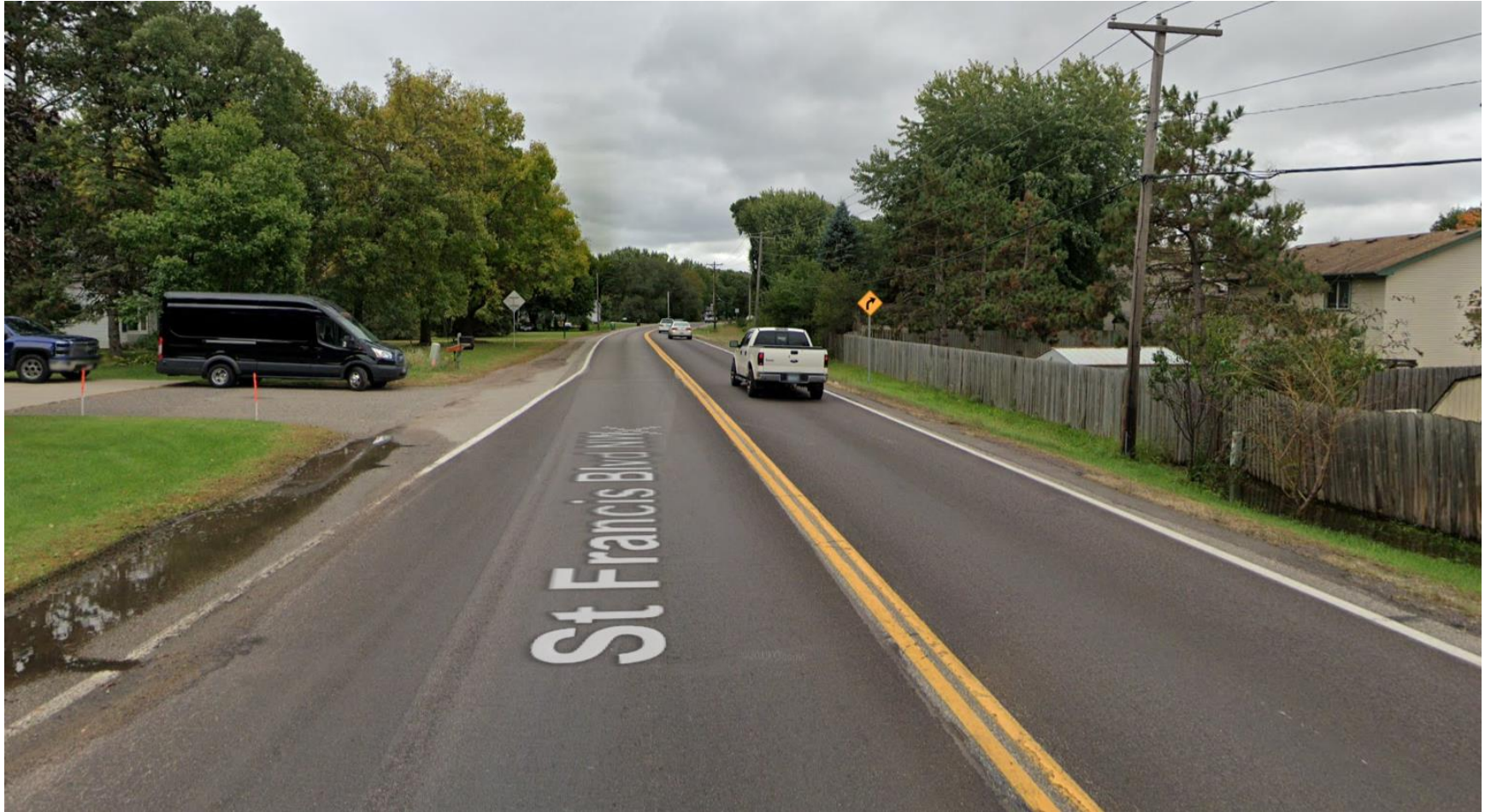
TH 47 Corridor Improvements – Existing Conditions: South of Coolidge Street, looking south
