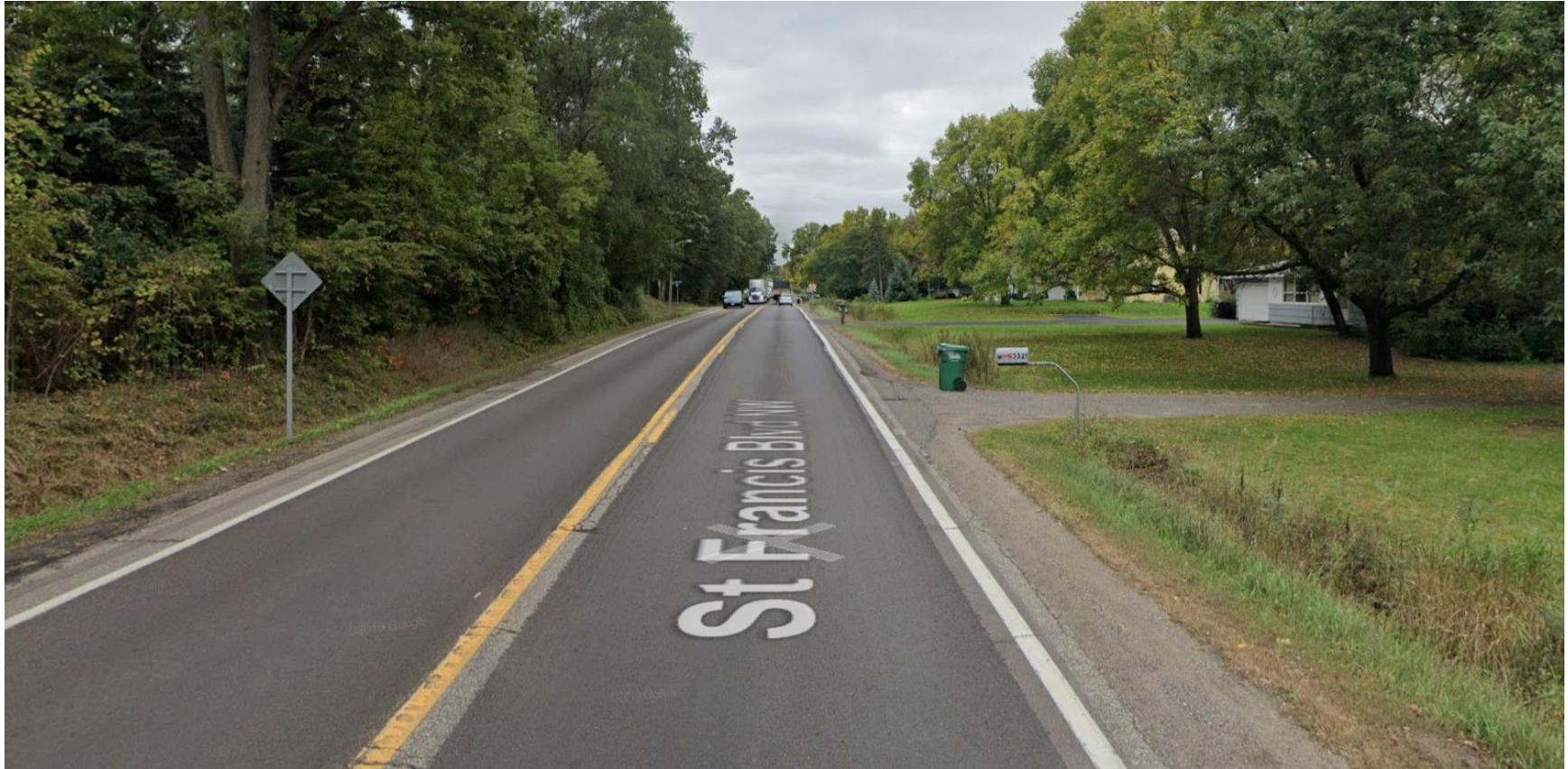
TH 47 Corridor Improvements – Existing Conditions: South of Dunham Drive, looking south
