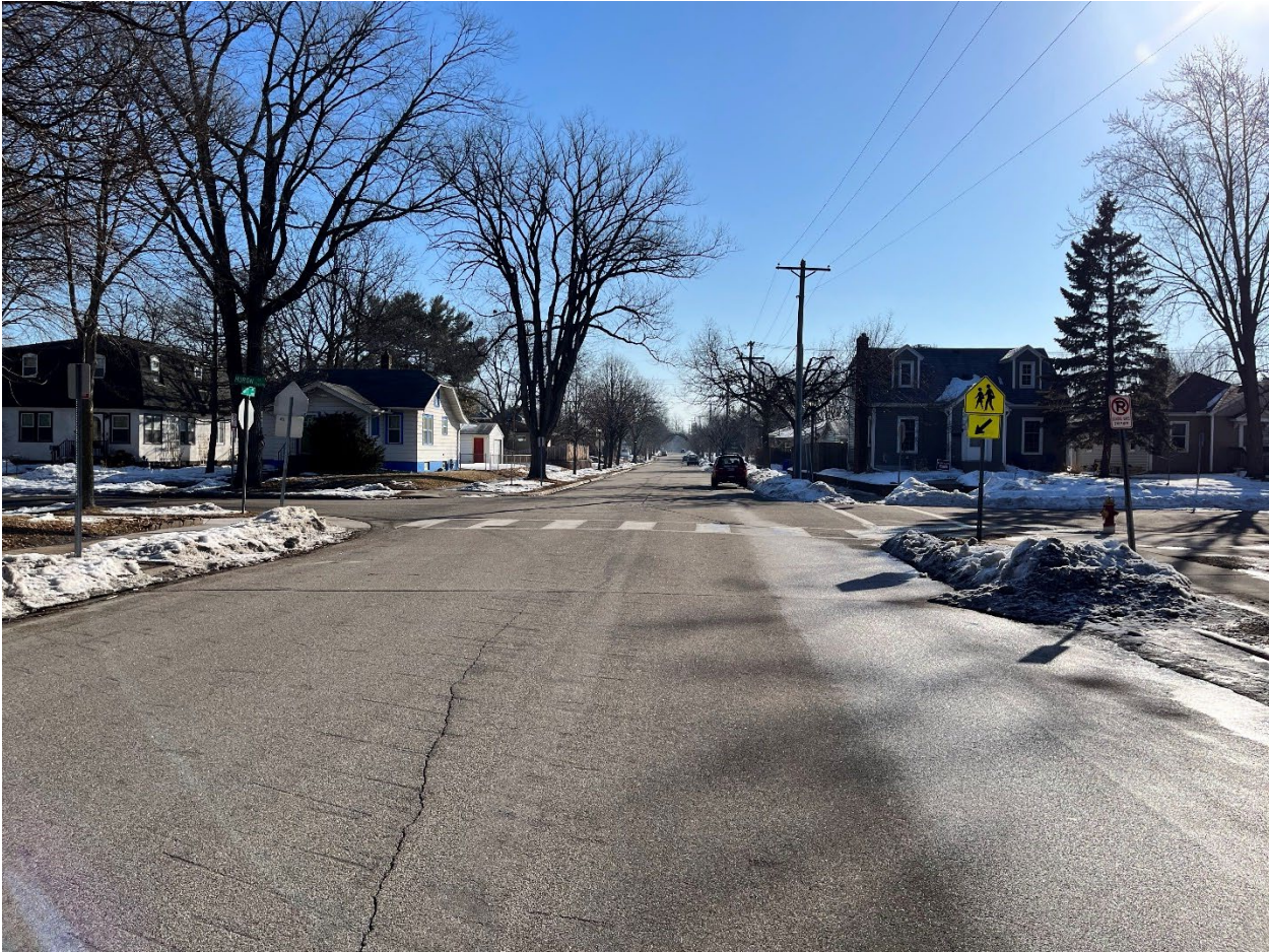
Hoyt Ave and Huron St - March 2022 (40 foot crossings)
