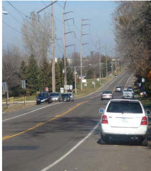
Roadway in Anoka County (Source: Anoka County)
