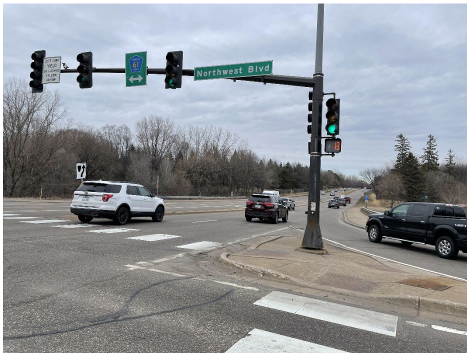
Eastern signal leg, originally constructed in 1987.
