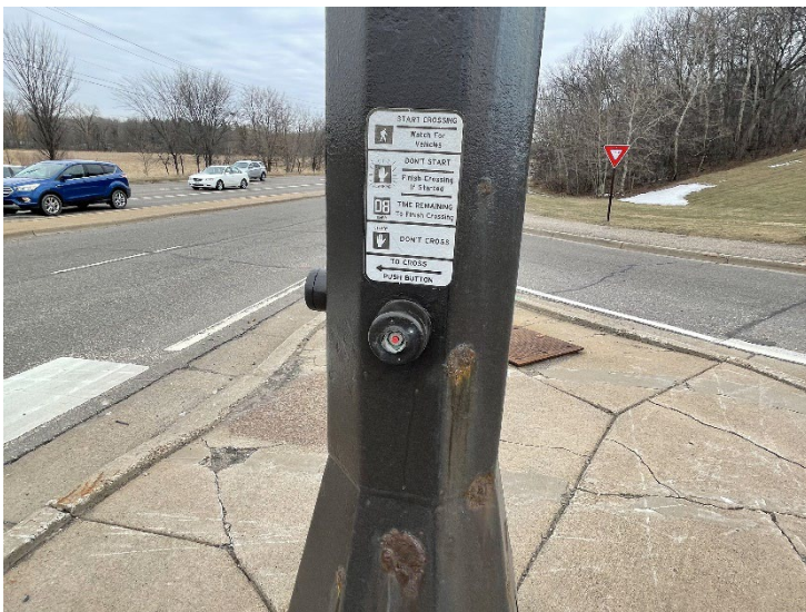
Aging Accessible Pedestrian Signal, southwest intersection quadrant.
