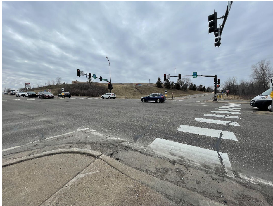
Eastern pedestrian crossing across CSAH 9.
