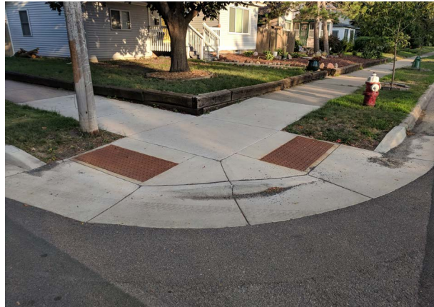
Figure 4-3: Combined Directional Ramp
