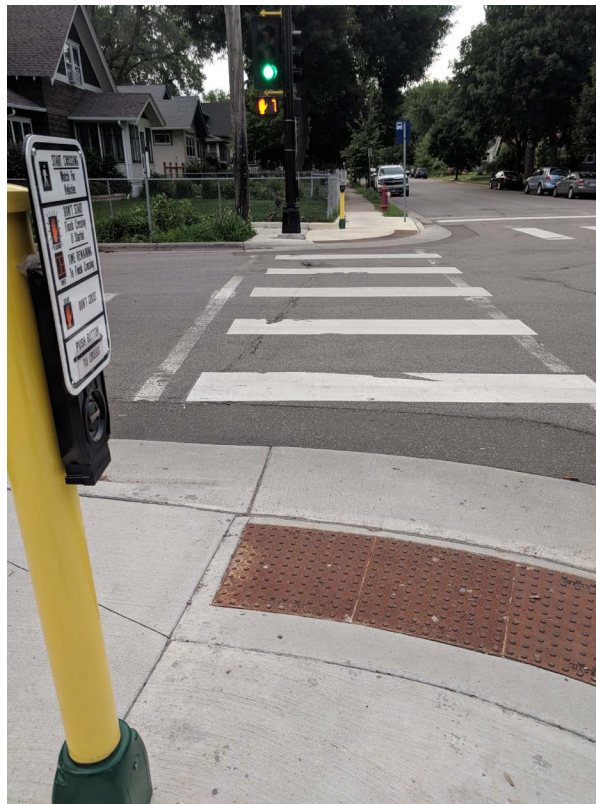
Figure 3-9: Push buttons and pedestrian signal heads are components of Accessible Pedestrian Signals (APS)
