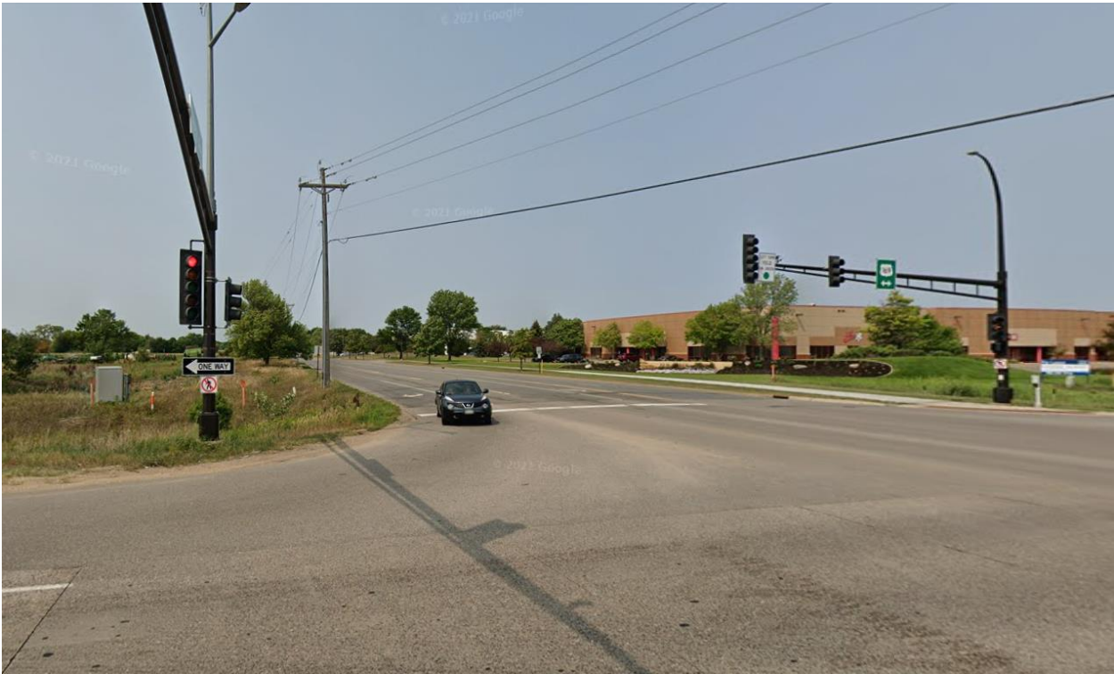
Photo 2: West Leg of US 169 and 109th Avenue N intersection (Aug 2021) Photo Credit: Google Street View
