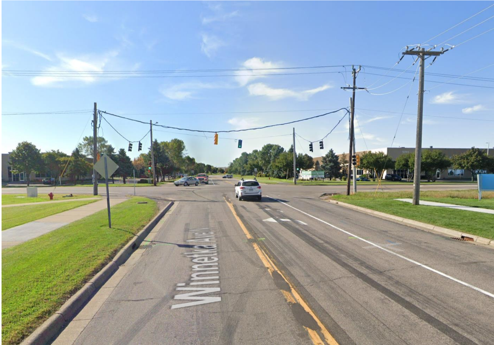
Winnetka Ave Existing Conditions – Looking south towards CSAH 30
