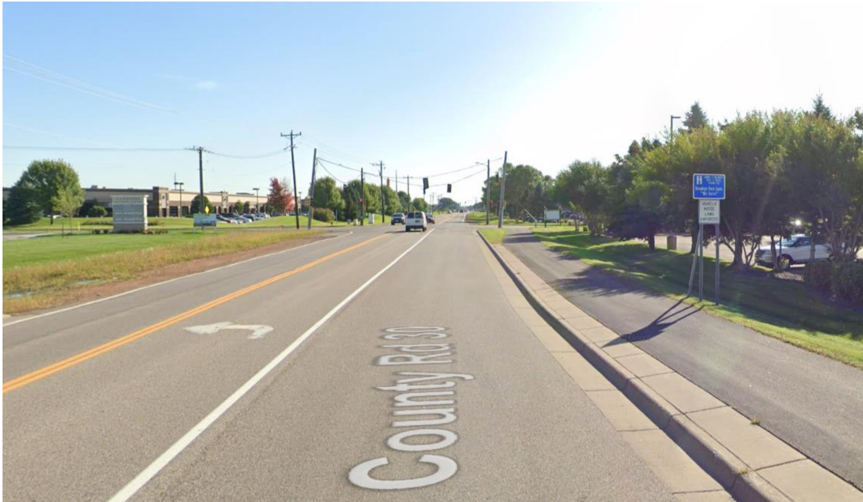
CSAH 30 Existing Conditions – Looking east towards Winnetka/Wyoming
