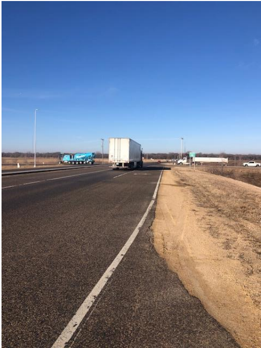
Looking west at CSAH 46/TH 52 interchange
