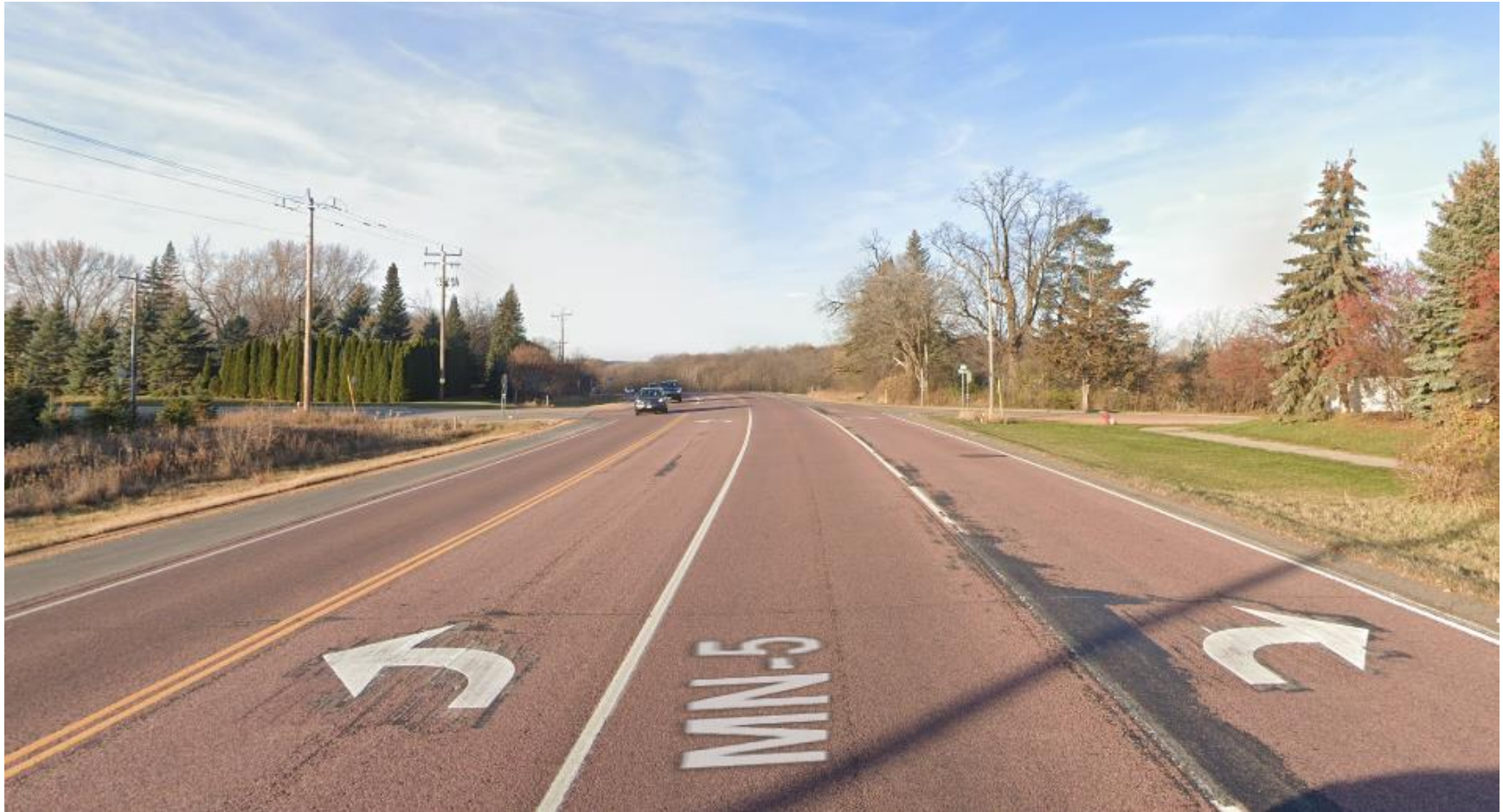
TH 5 at Kochia Lane/Park Dr Existing Conditions – looking west
