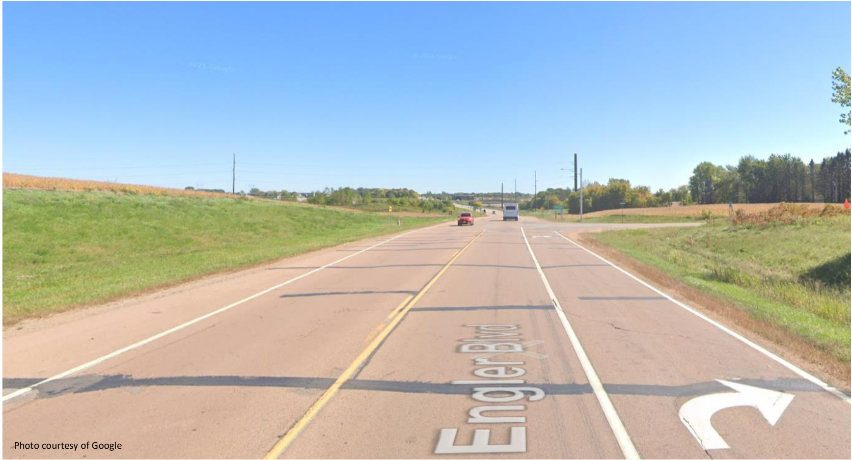
CSAH 10 at Creek Road Intersection Existing Conditions – Looking east
