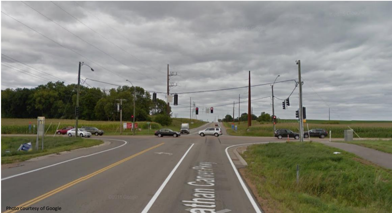
CSAH 10 at CSAH 11 Intersection Existing Conditions – Looking north
