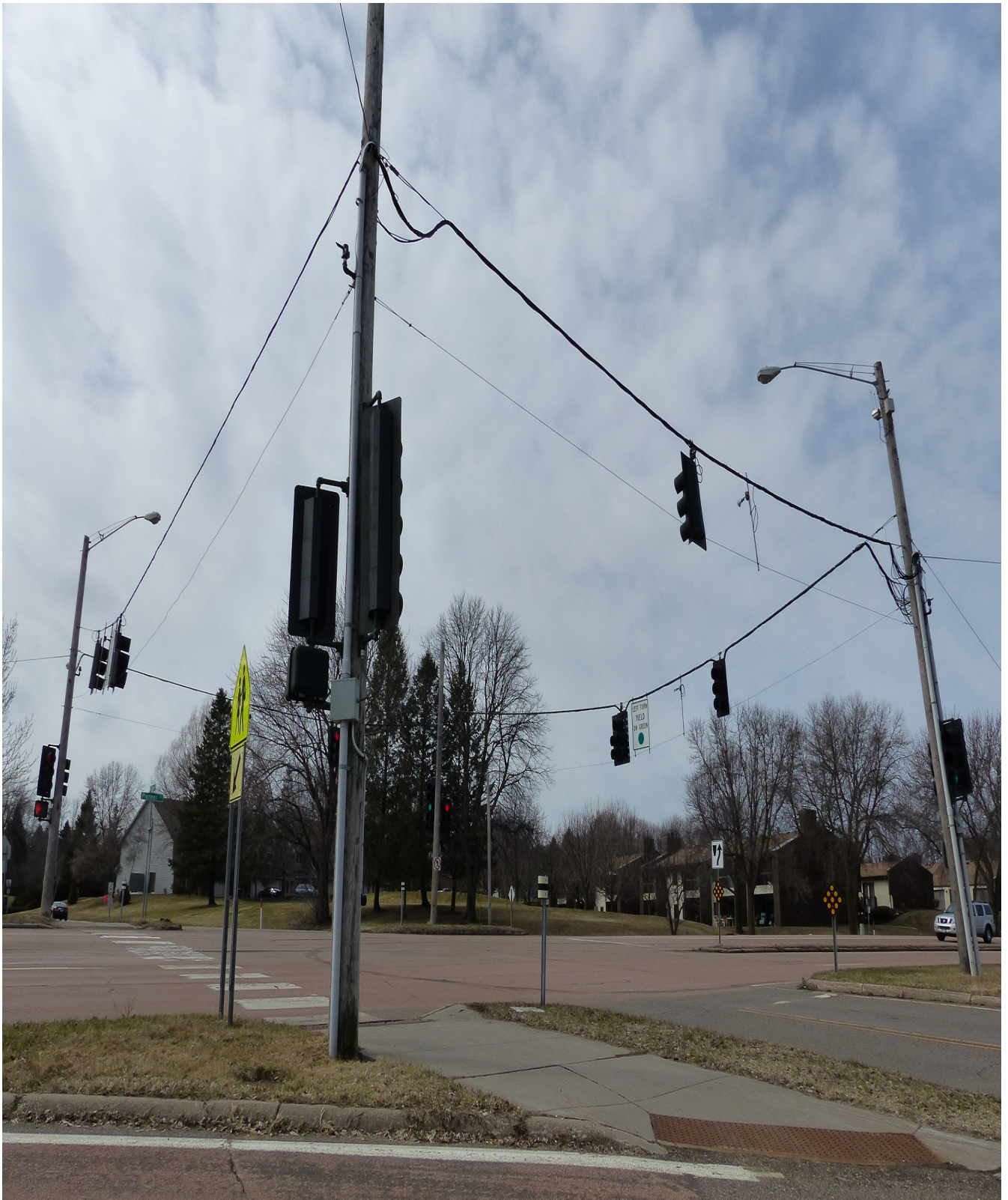
Carver County photograph showing the existing conditions within the project area.
