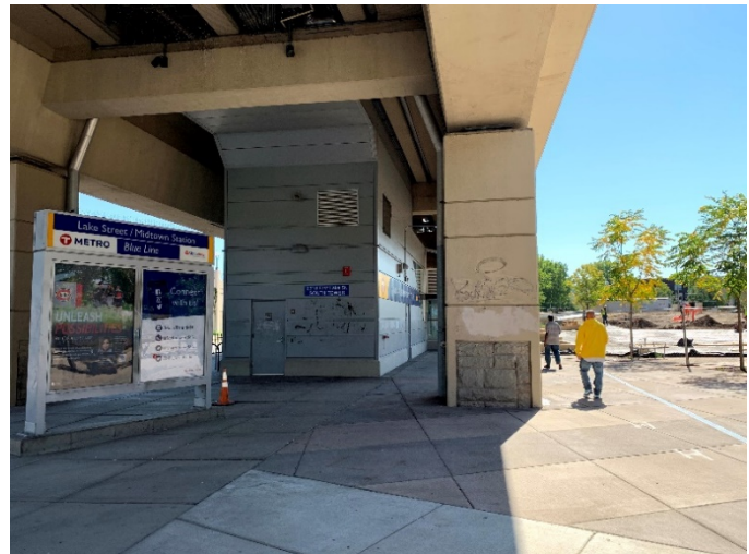
Approach of the South Tower from Lake Street
