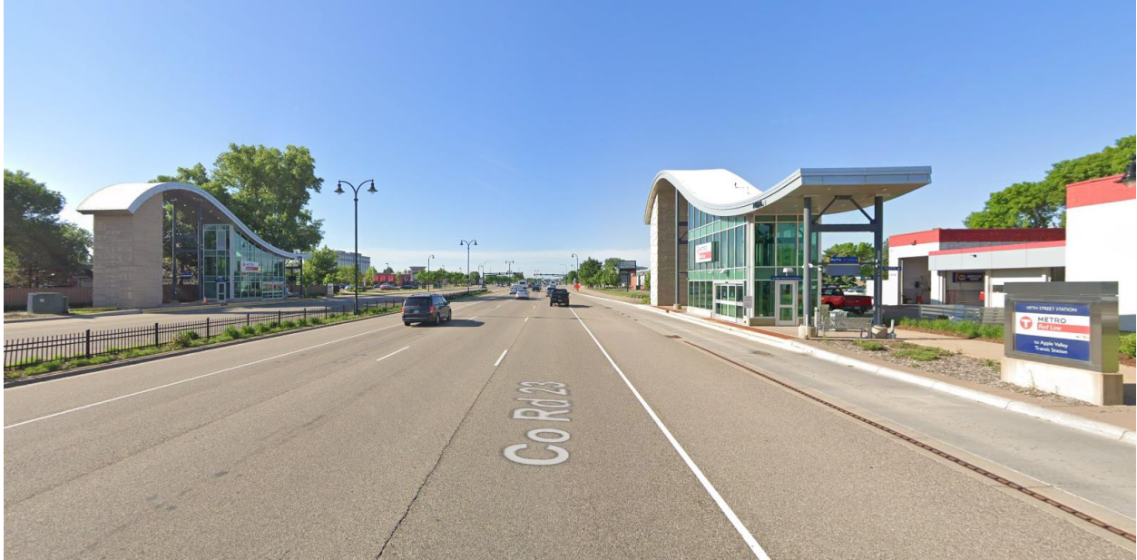
Existing Conditions: Cedar Avenue southbound, approaching 147 th Street Station
