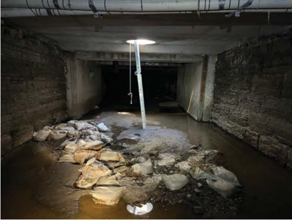
General northward view of Basset Creek under CSAH 40 (Glenwood Ave).
