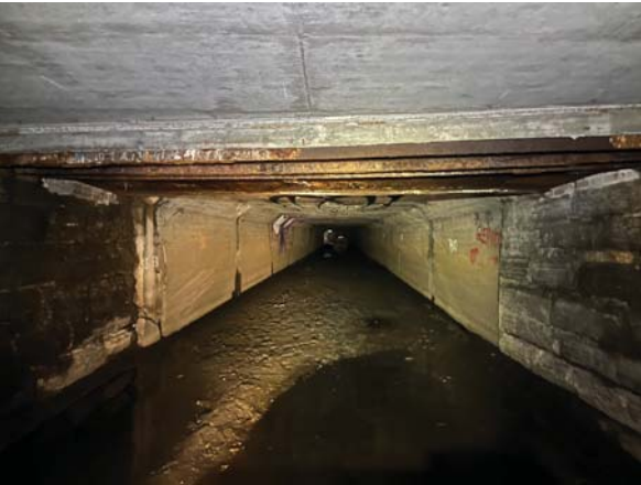
General view of south approach.
