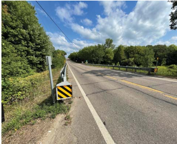
View of Fernbrook Ln (CSAH 121) roadway conditions pictured above.
