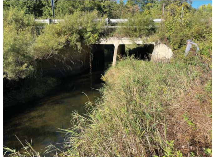
East elevation of the bridge is pictured above.
