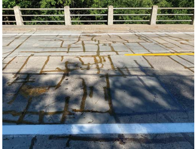
Patches and sealed cracks on the bridge deck.
