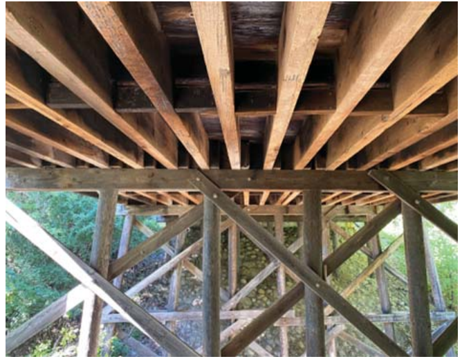
Timber framed substructure and superstructure.
