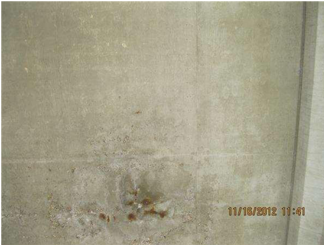
Photo 22 - rebar on deck bottom2
