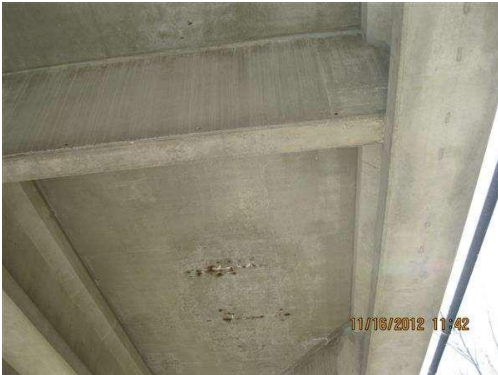
Photo 25 - rebar on deck bottom5
