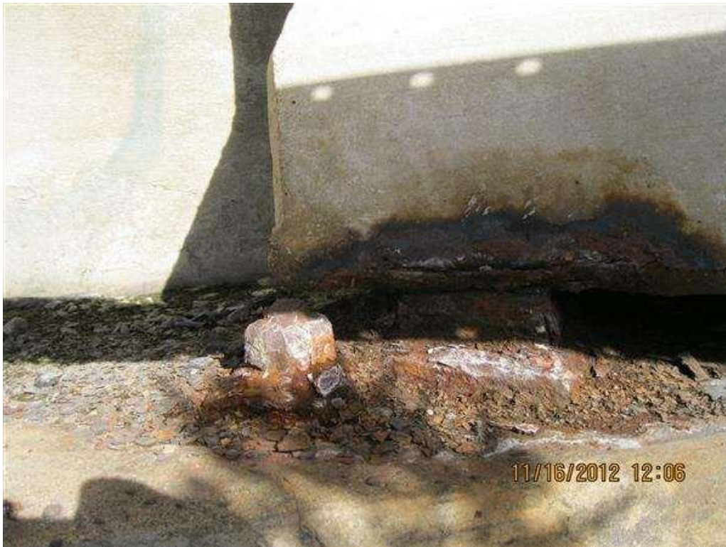
Photo 12 - corroded bearing
