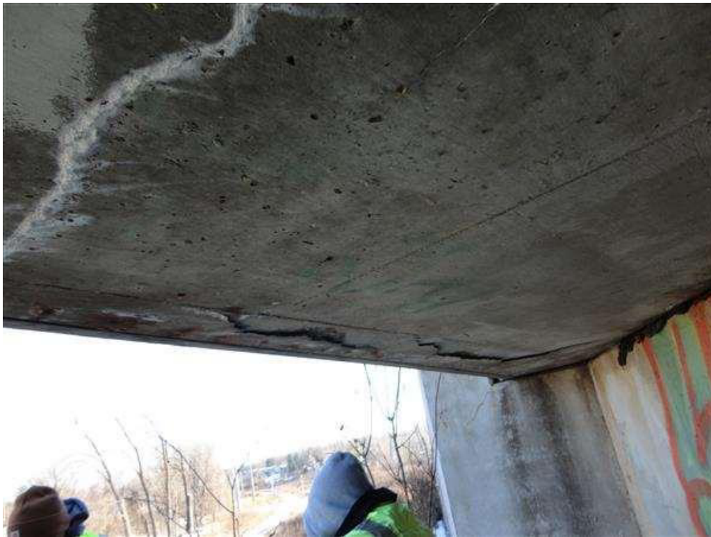
Photo 4 - delamination on SW corner
