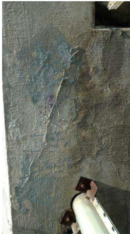
Photo 31 - SW Abutment diagonal crack 2018
