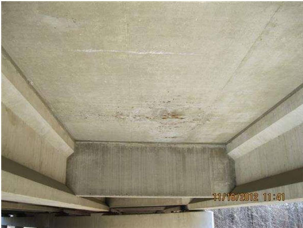
Photo 21 - rebar on deck bottom
