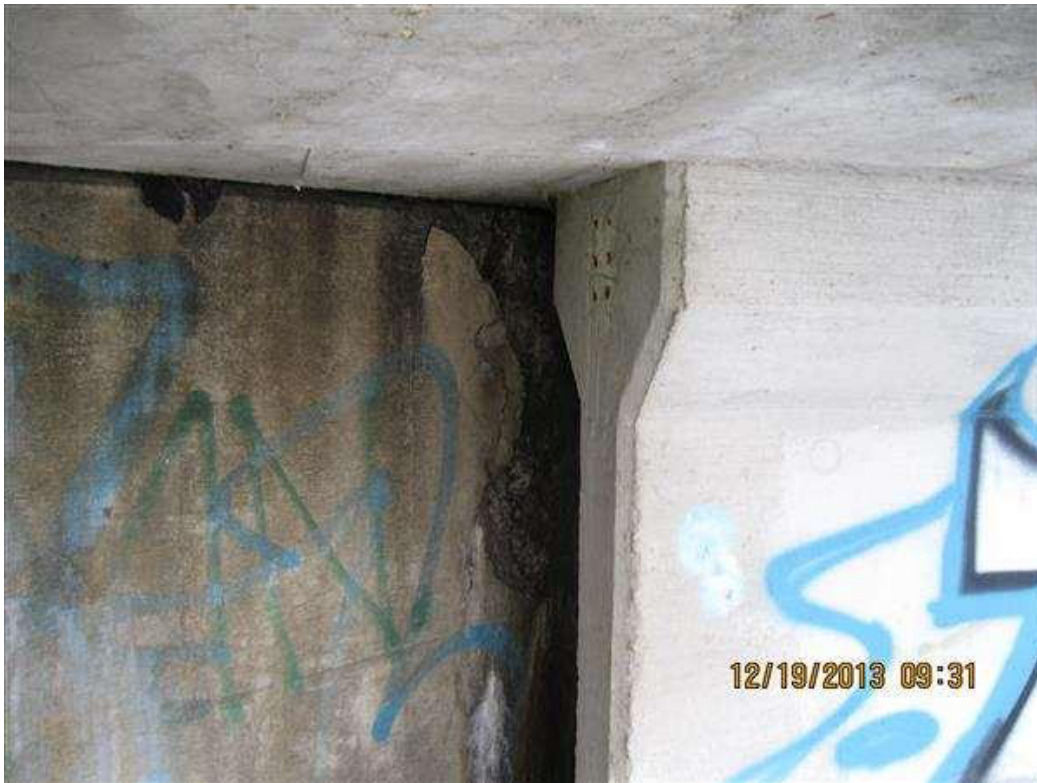
Photo 26 - Spall in S. corner 2013
