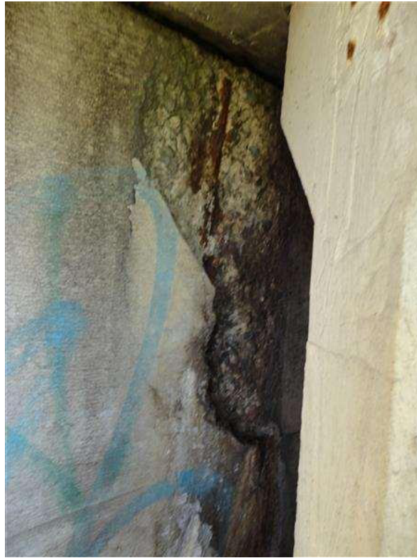
Photo 7 - spall on SW corner parapet
