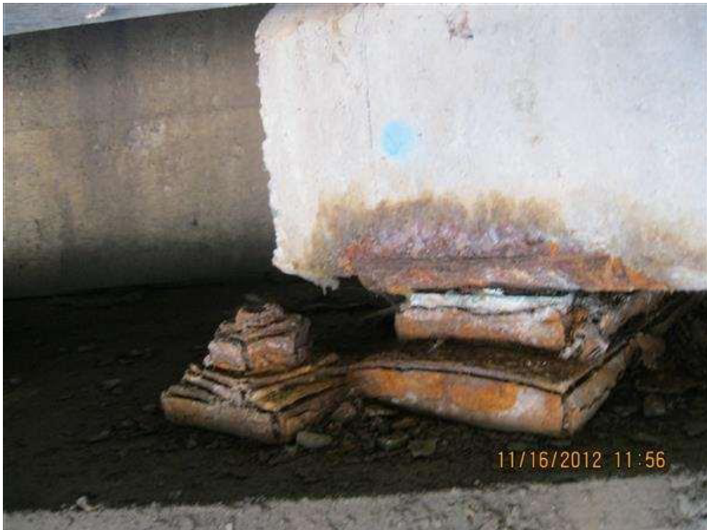
Photo 10 - bearing on southwest corner
