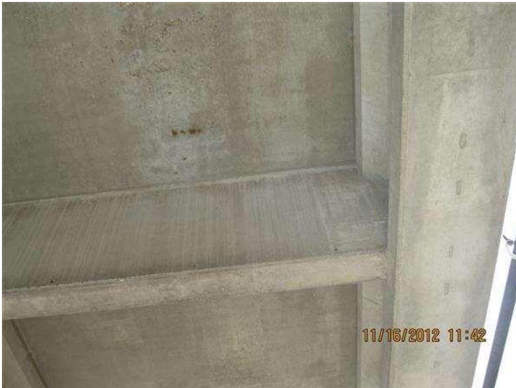
Photo 23 - rebar on deck bottom3
