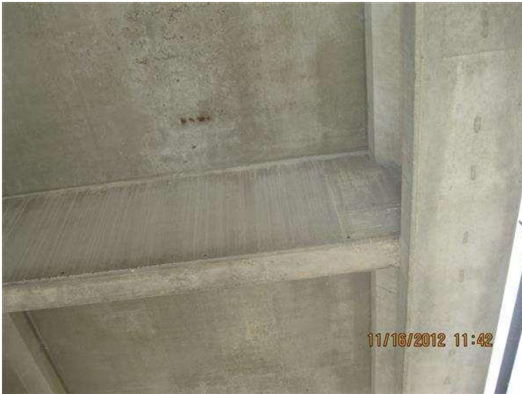
Photo 24 - rebar on deck bottom4
