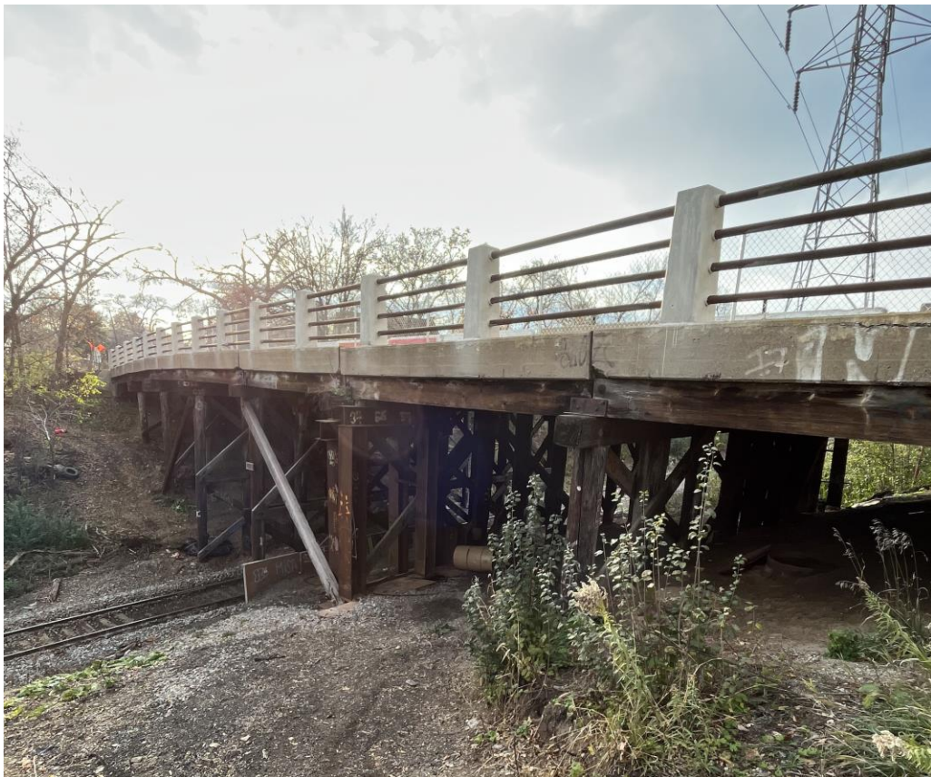
Cedar Lake Road Bridge Elevation View Looking SW
