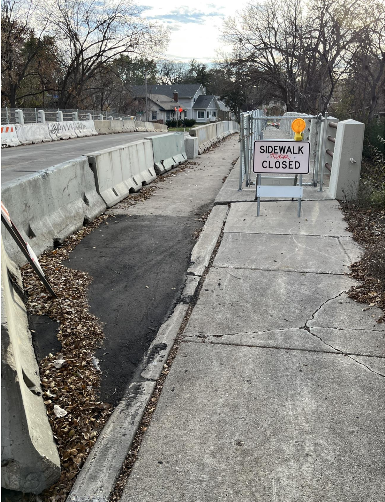
Sidewalk Closure – Temp Relocation onto Bridge Deck
