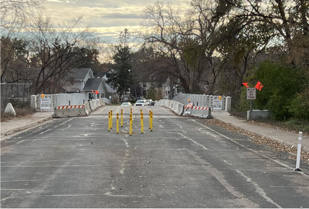
Cedar Lake Road Looking SW
