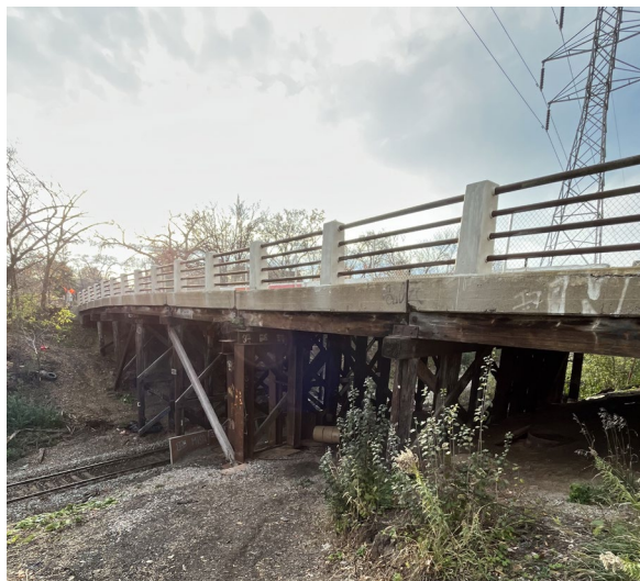
Cedar Lake Road Bridge 90471 over BNSF RR
