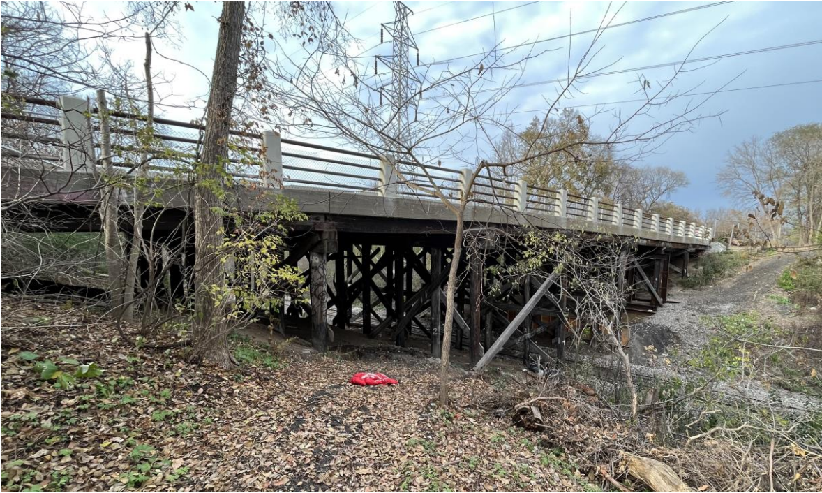
Cedar Lake Road Bridge Elevation View Looking NE
