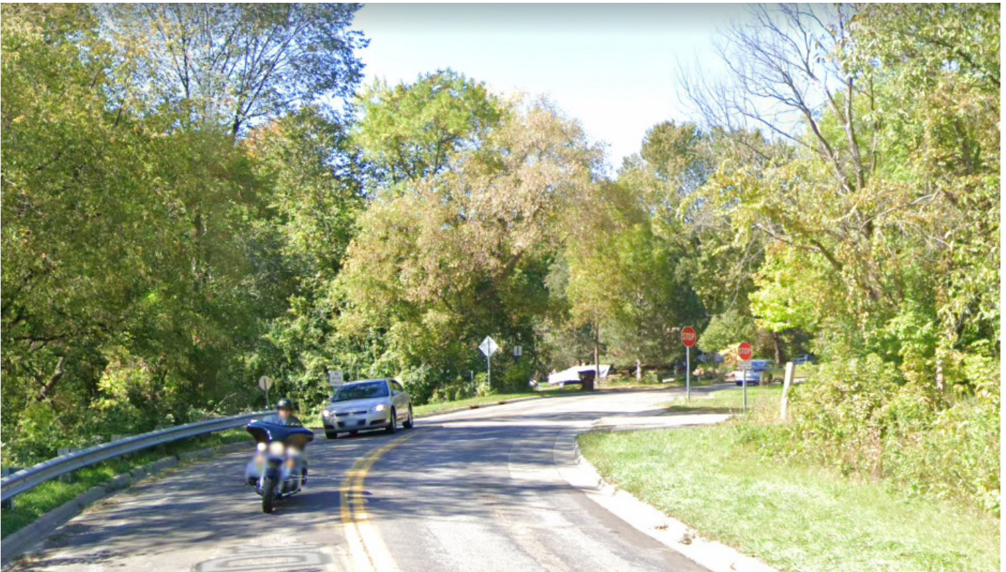
Unsafe trail crossing; limited sightlines and signage (looking northwest)
