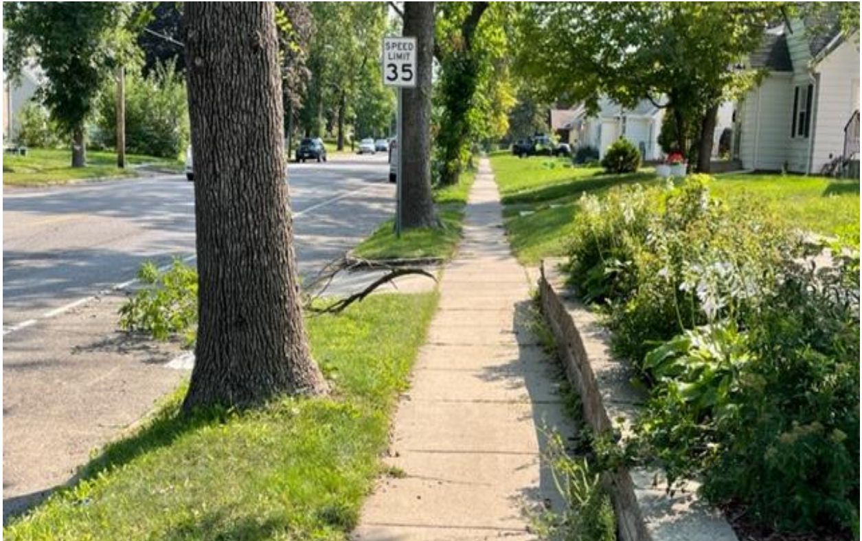
Figure 4: Existing conditions on Butler Ave, between Oakdale Ave and Carrie Street.
