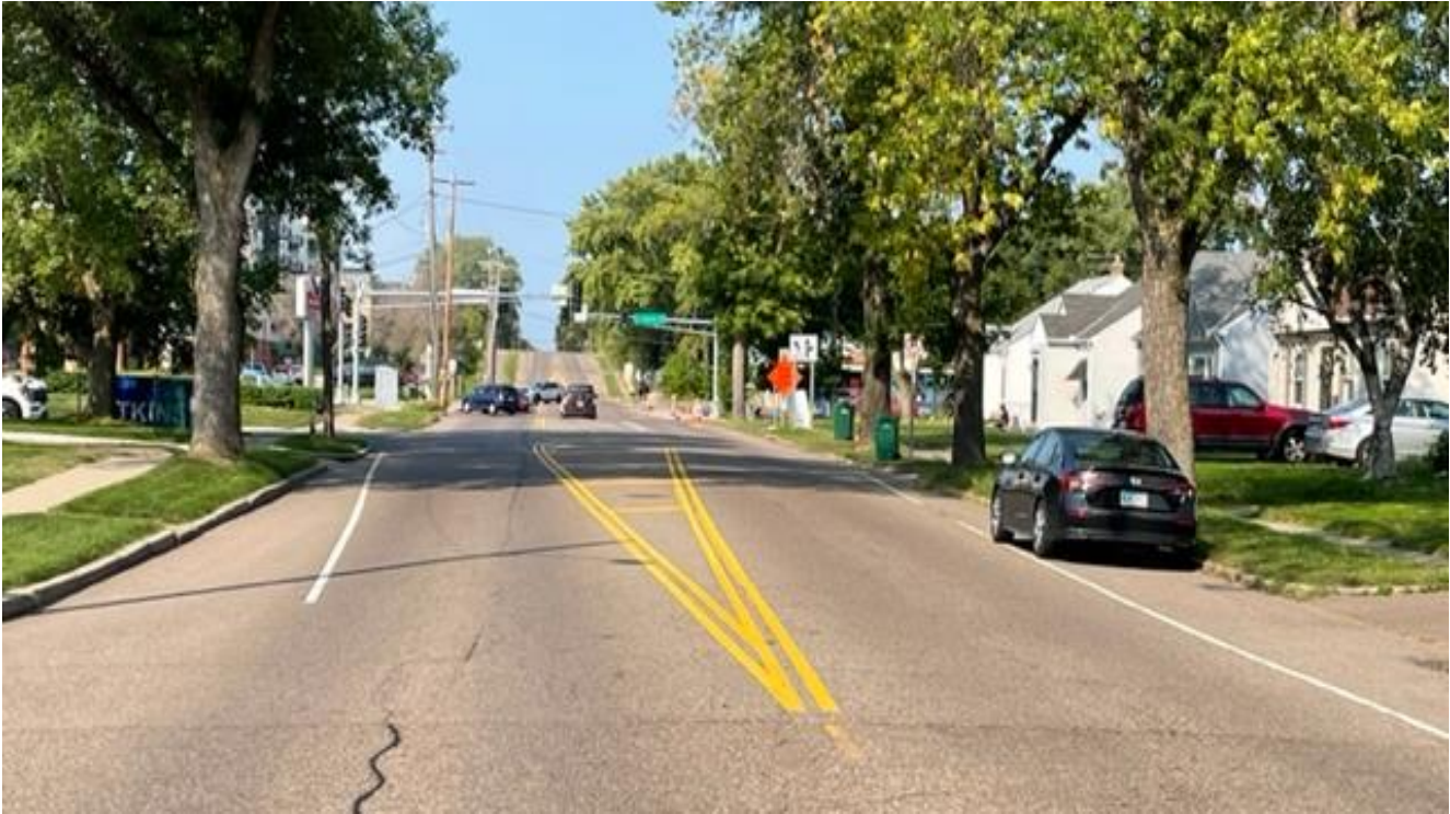
Figure 2: Existing conditions on Butler Ave, between Westchester Place and Kruse Street.
