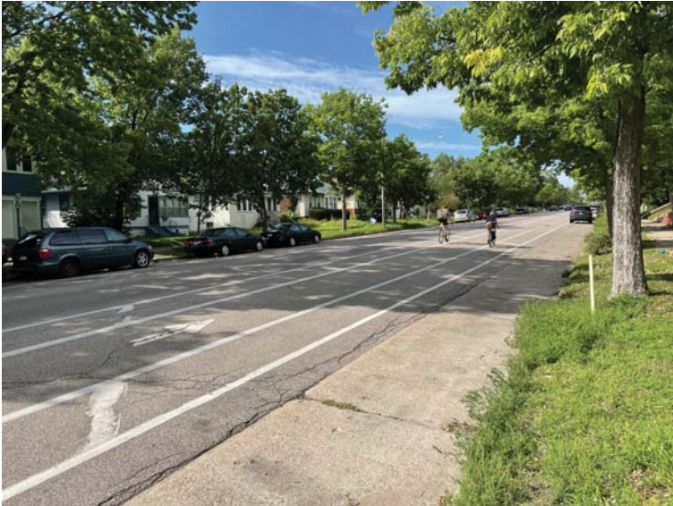
The current infrastructure for people biking lacks separation from parked vehicles and people driving.
