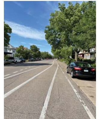
Park Ave (CSAH 33) existing bike infrastructure pictured.
