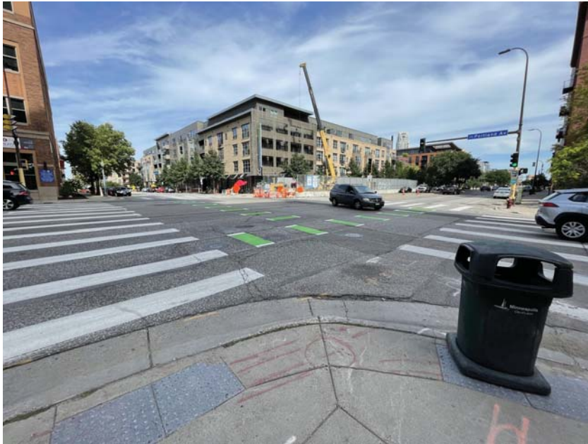
The Intersection of Washington Ave (CSAH 152) and Portland Ave (CSAH 35) is pictured above. Intersection signals pictured above are from 1957 and require replacement.
