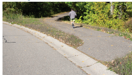
42nd Place North (left photo) and Northwest Blvd (CSAH 61) (right photo): This trail segment is missing critical ADA improvements (i.e. compliant curb ramps and truncated domes) and is comprised of failing pavement as shown by "alligator cracking" and patching. Pavement is no longer conducive to any pavement treatment and requires complete reconstruction.
