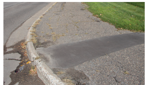
42nd Place North (left photo) and Northwest Blvd (CSAH 61) (right photo): This trail segment is missing critical ADA improvements (i.e. compliant curb ramps and truncated domes) and is comprised of failing pavement as shown by "alligator cracking" and patching. Pavement is no longer conducive to any pavement treatment and requires complete reconstruction.
