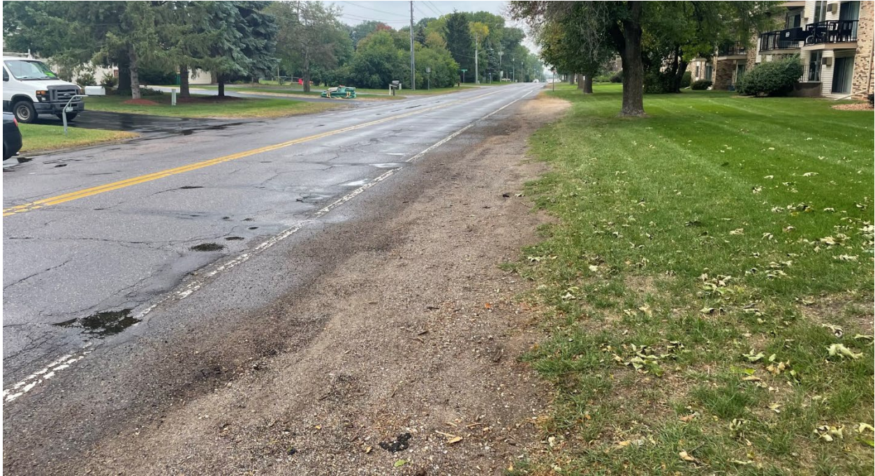
Figure 1 – Evidence of roadway condition
