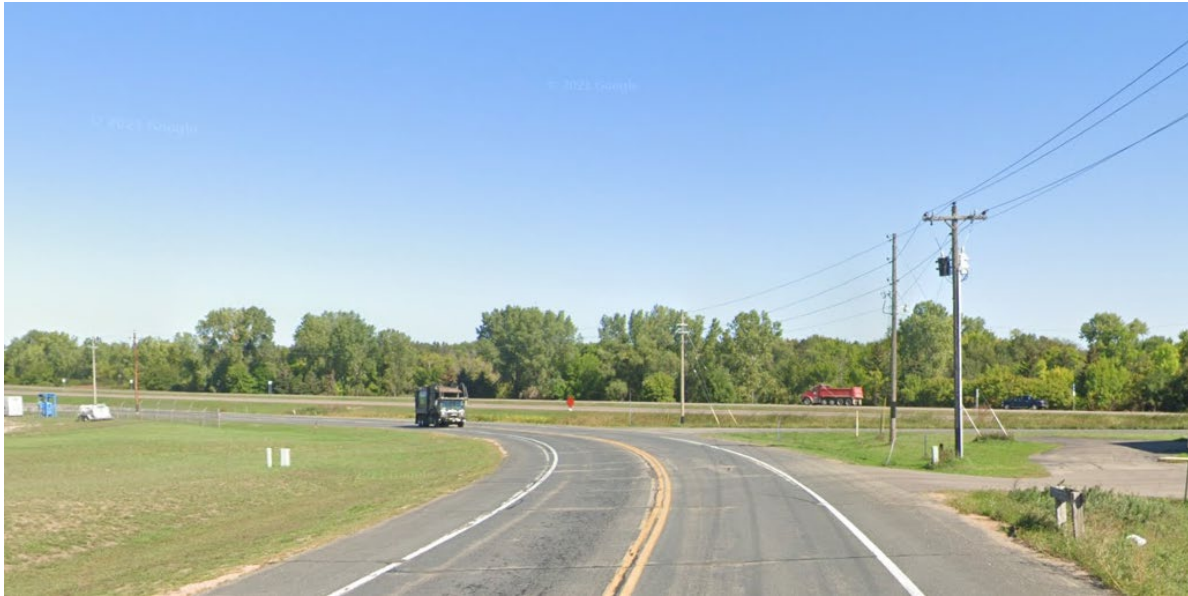
Figure 1: The horizontal curve in the roadway can create safety and visibility challenges with pedestrians walking on the shoulder.
