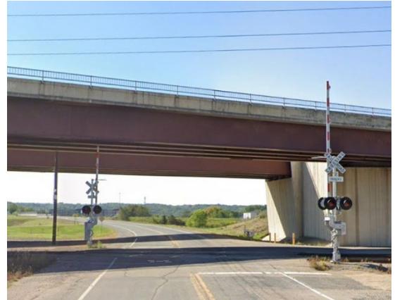
Existing conditions along Stagecoach Rd
