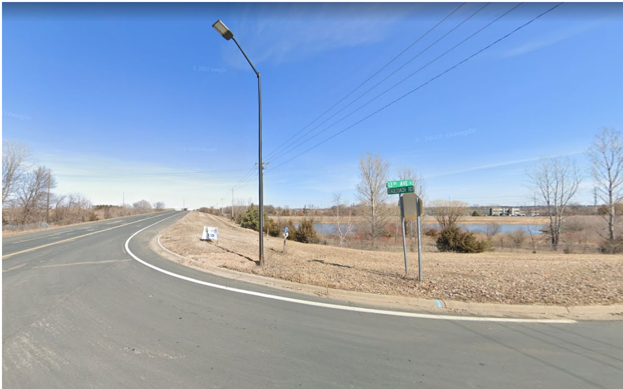
Figure 6: The southern end of the corridor at Stagecoach Rd and 13th Ave.
