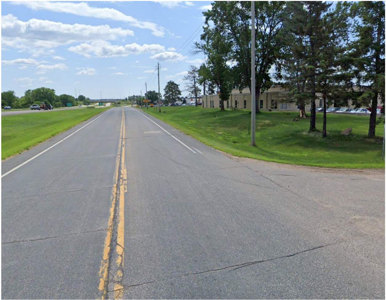
Figure 3: Narrow shoulders and drainage ditches along Stagecoach Rd.
