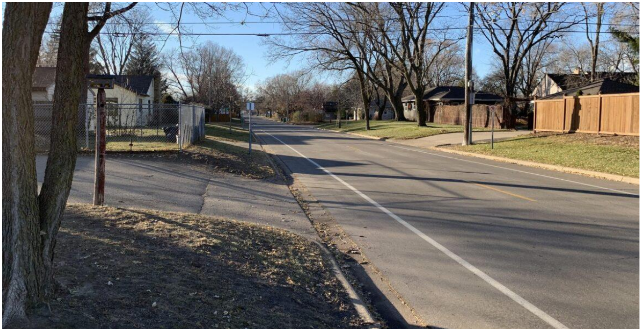
Photo 4: 64th St near 3rd Ave S, facing west (Nov 2023). Photo Credit: City of Richfield
