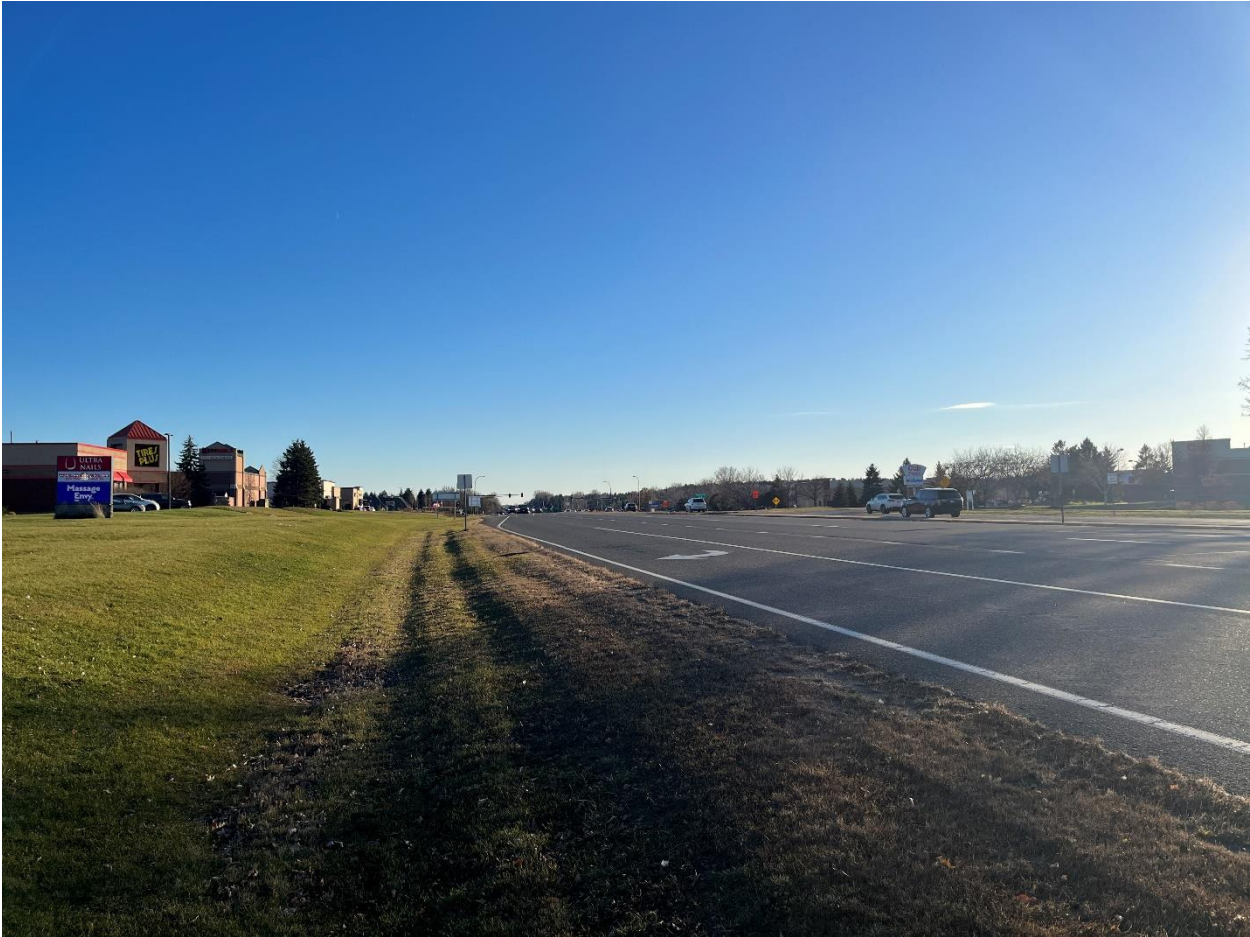
East side of Radio Drive at Hudson Road facing south
