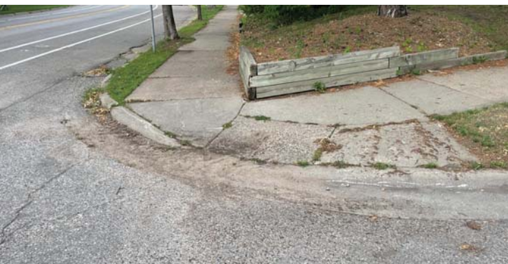
Many ramps along Portland Ave (CSAH 35) lack ADA compliant truncated domes and need repair. The pictures above highlight non-compliant pedestrian infrastructure at the 53rd St intersection.
