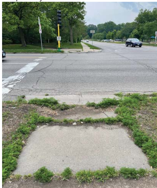
Many ramps along Portland Ave (CSAH 35) lack ADA compliant truncated domes and need repair. The pictures above highlight non-compliant pedestrian infrastructure at the 53rd St intersection.
