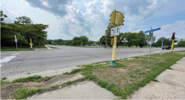
The intersection of Portland Ave (CSAH 35) and E Diamond Lake Rd is pictured above. The signal system was constructed in 1960 and requires replacement.
